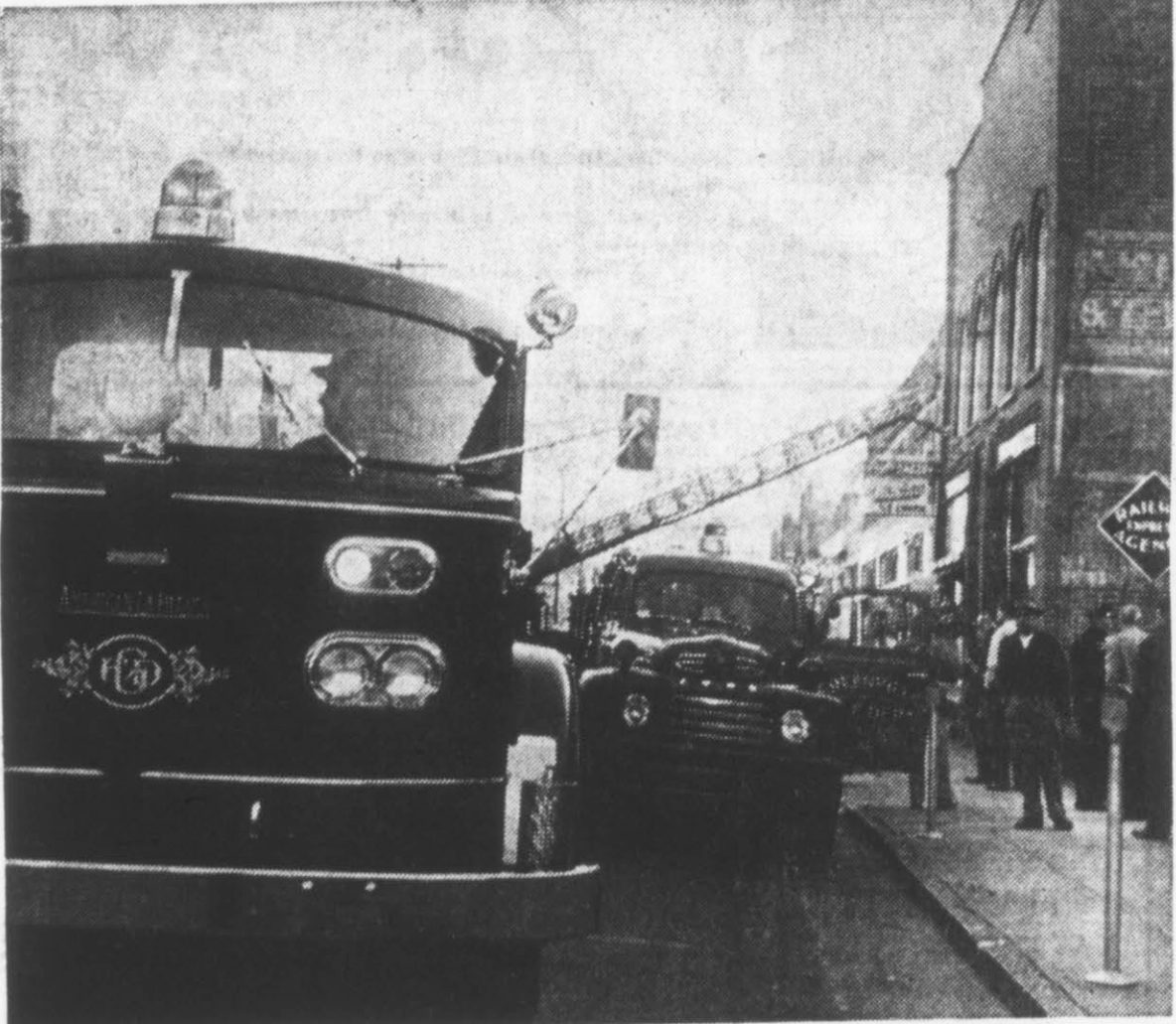
SMOKE SCARE . . . Greenville fire trucks are shown stopped on Dickinson Ave. early today as firemen checked for a fire in the Diener's Bakery-Railway Express building in the 800 block of Dickinson. Firemen were called to the scene about 7:01 a.m. when smoke was reported coming from the structure. Fire alarm box 122, at the intersection of Dickinson Ave. and Clark St. was turned in for the "fire." In a call yesterday, local firefighters extinguished a blaze in a car owned by George Howard, Jr., which caught fire at the intersection of Ninth and Washington Sts. about 6:55 p.m. Damage to the vehicle's carburetor was reported.
