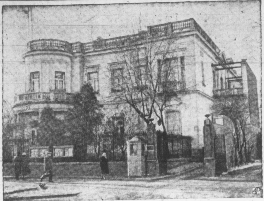
EMBASSY IN WARSAW —This old structure on Wjazdowski Street houses the United States embassy in the downtown section of the Polish capital. Construction work has started on a new building to provide more modern quarters for the American delegation.
