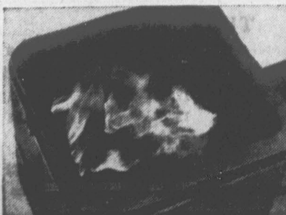
Old-fashioned heating oil may form deposits that can choke the nozzle openings of the burner, producing an unbalanced flame. Heat bills can run high.
