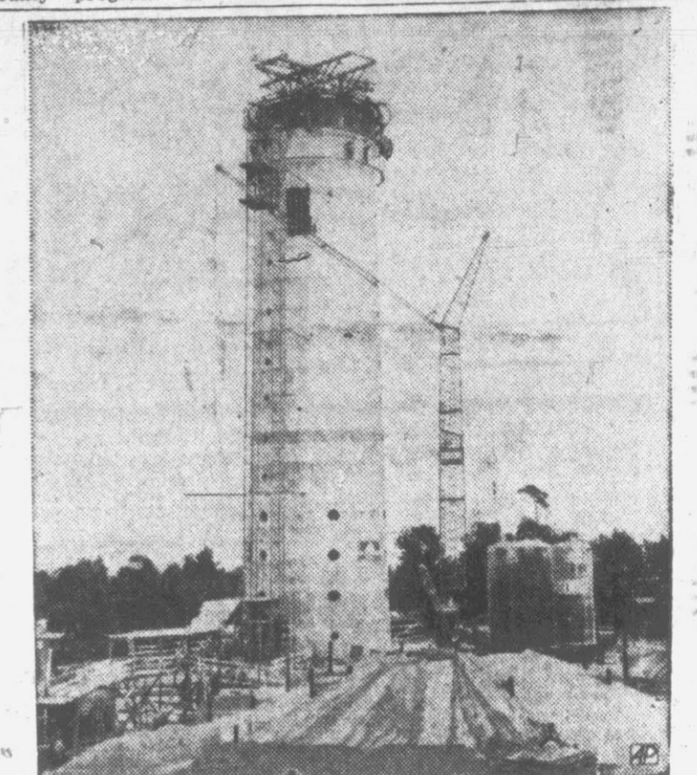
GERMAN LINK — A 895-foot high TV tower rises in Wannsee area of Berlin. It will serve radio-telephone communications between Berlin and West Germany.
