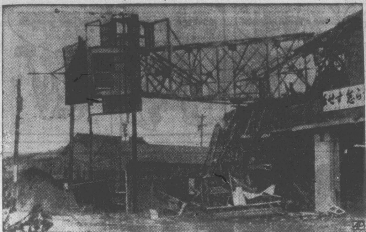
TYPHOON NANCY LASHES JAPAN —This steel fire observation tower was broken in half as Typhoon Nancy slammed into Osaka, second largest city in Japan. The giant Pacificborn storm damaged or destroyed thousands of homes, leaving scores dead, missing and injured. (AP Wirephoto by radio from Tokyo)
