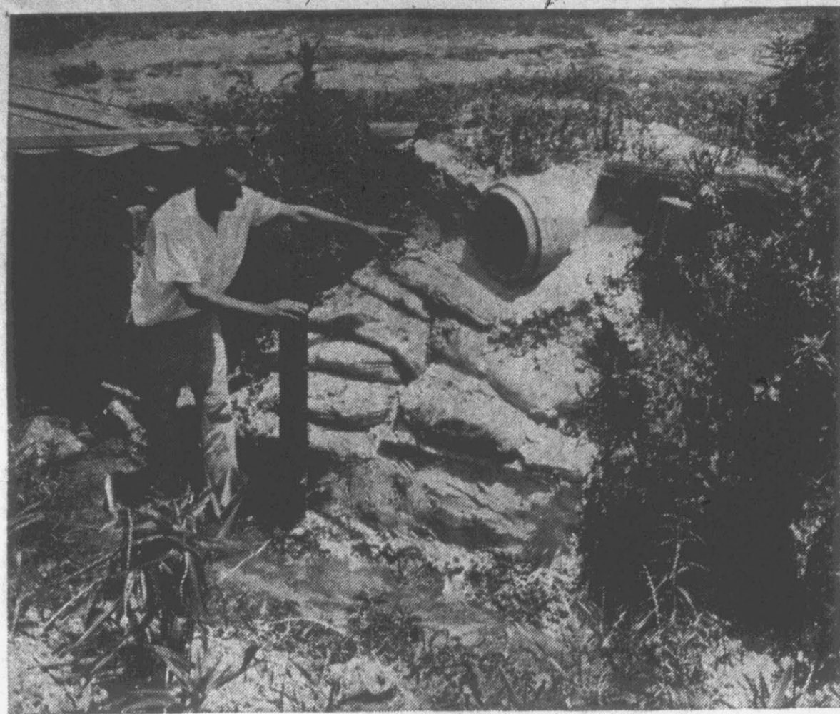
EROSION CONTROL —Soil Conservation Service aide Elmer Bland here points to a masonry overfall and surface inlet installed by Harry J. Byers on his farm near Bell Arthur. "This structure will prevent a gully from developing in the side of this main drainage ditch," Bland says of the installation. Technical assistance in this and other phases of conservation planning is made available to landowners in the Pitt area through the Coastal Plain Soil and Water Conservation District. Farmers may apply for such help to district supervisors. Arch J. Flanagan of Farmville, W. C. House of Bethel or Brantley Speight of Winterville. (SCS Photo by Roy R. Beck)
