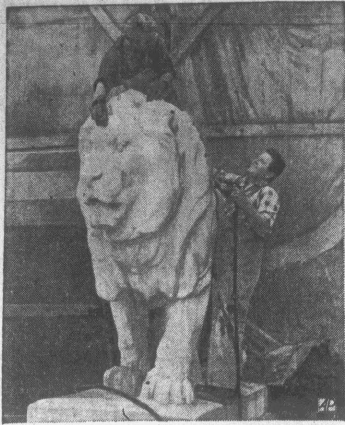
SCRUB 'N BLAST —Workmen clean stone lion at the Feldherrnhalle in Munich as the Bavarian capital's monuments and historic buildings undergo a facelift.
