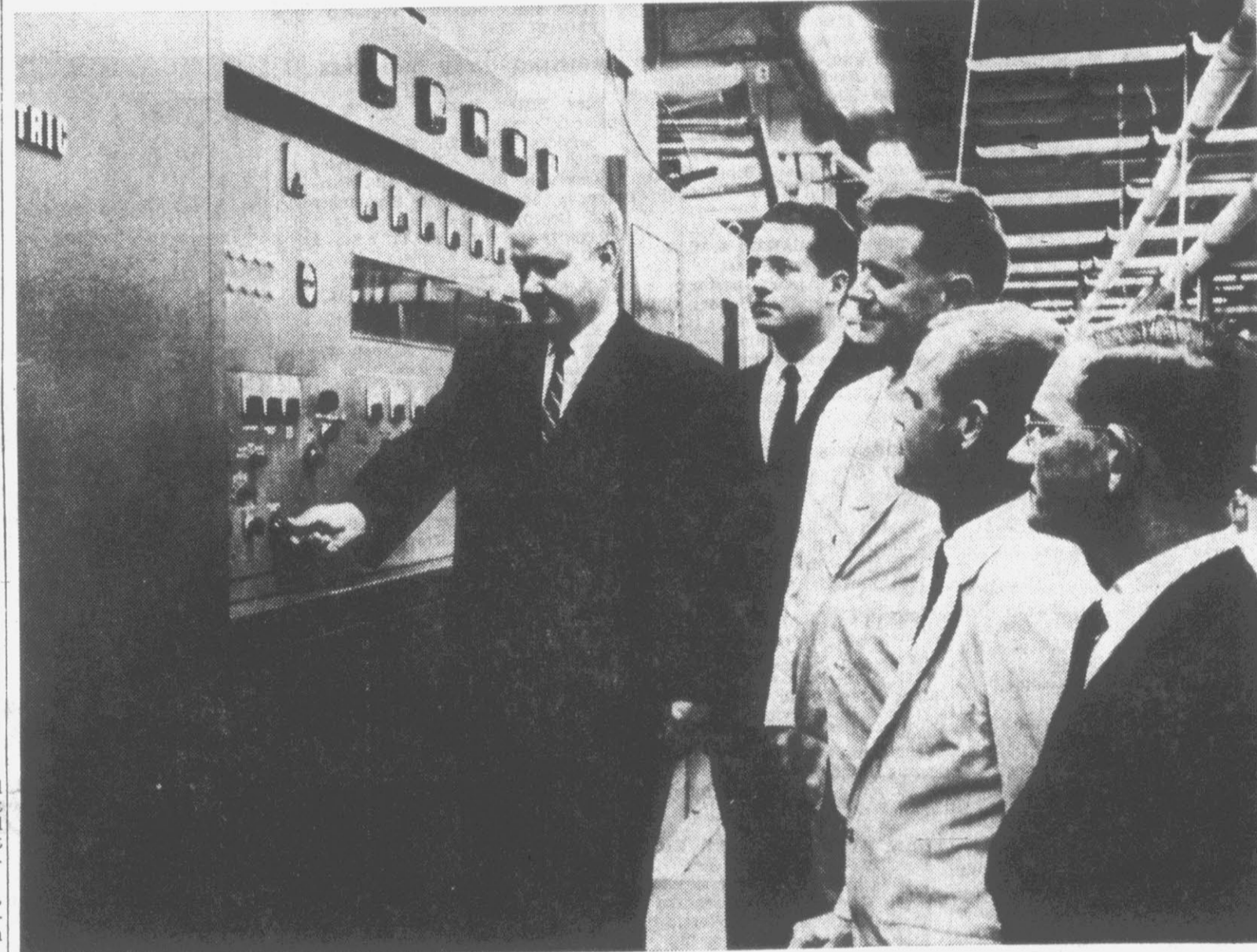
GIVING AMERICA A STRONGER VOICE—United States Information Agency officials view General Electric super-power short-wave radio transmitter built for Voice of America's consolidated East Coast facility near Greenville. Robert L. Casselberry (left), general manager of the Company's Technical Products Operation, which designed and manufactured the 250,000-watt unit, describes its features during inspection tour at G-E's Electronics Park, Syracuse, N.Y., where USA accepted transmitter. Others (left to right) are John W. Stonig, G-E sales engineer, and Paul Lee, W. R. Harmon and C. J. Affelder, all of USA. This one of 12 of these powerful transmitters General Electric is building for the Voice—six for Greenville and six for new installation near Monrovia, Liberia, on the west coast of Africa. Transmitters are equipped with special electronic devices to give them maximum effectiveness in beaming Voice of America broadcast signals throughout the world.
