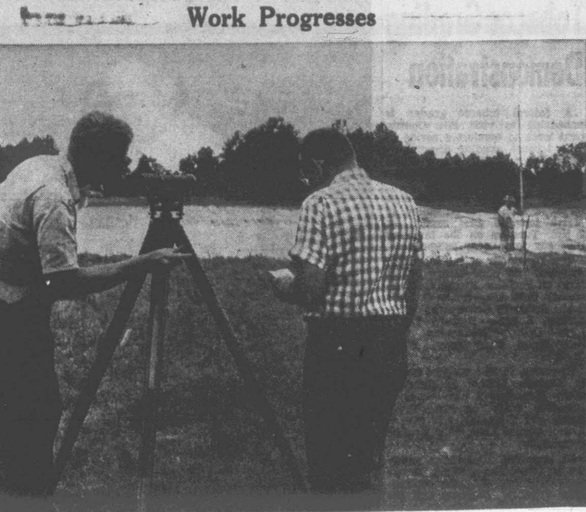
ENGINEERS surveying and leveling the new athletic facilities under construction at East Carolina College. (Reflector Staff Photo)
