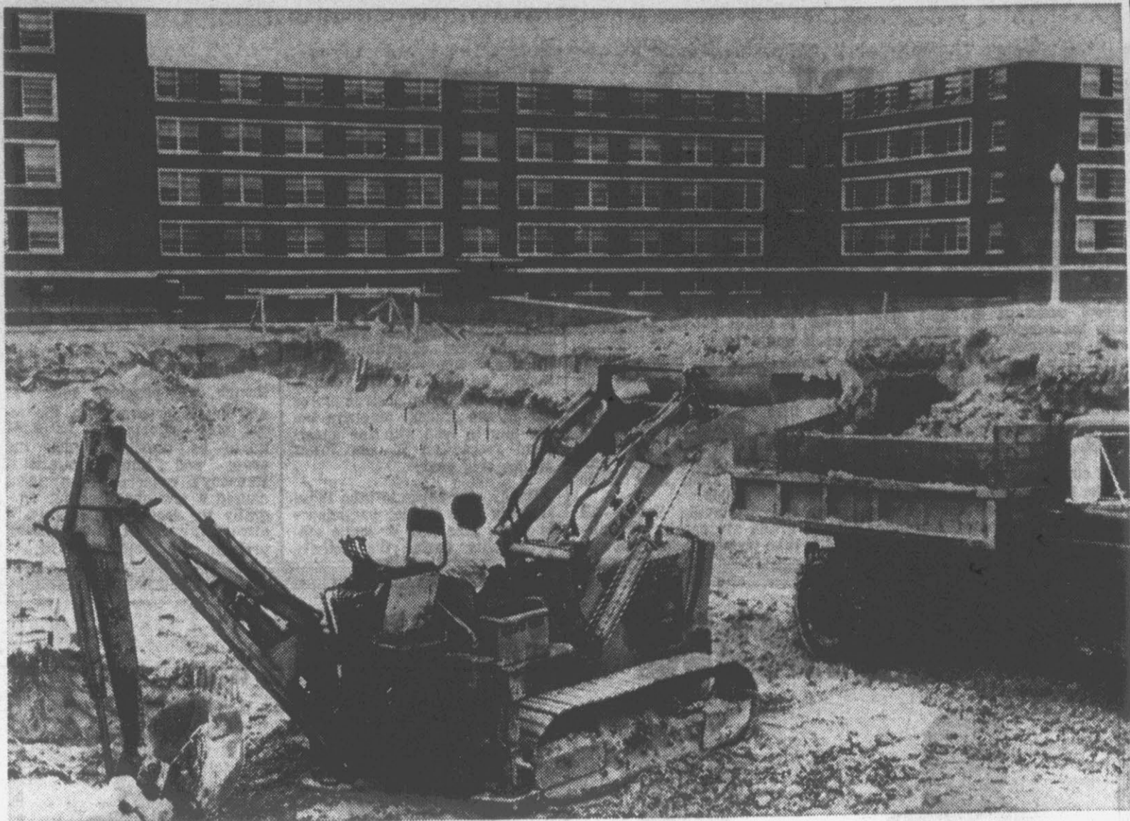
NOW UNDER CONSTRUCTION . . . Work has begun on a third 500-man dormitory on East Carolina College's South Campus. The structure will cost an average of $2,310 per student, with total cost set at $1,155,114. Completion date for the four-story building is scheduled for August 15, 1962. The new dorm, varying in design from Jones and "A" dormitories, will include outside corridors on each floor with outside entrances to four-room suites. Excavation is shown here with "A" dorm in the background. (Reflector Photo by Stuart Savage)
