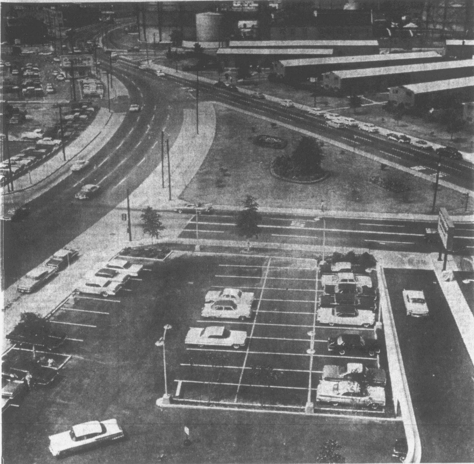
OFF STREET PARKING AND ADEQUATE STREETS . . . characterize Norfolk's urban renewal. Seven thousand parking spaces will be provided.
