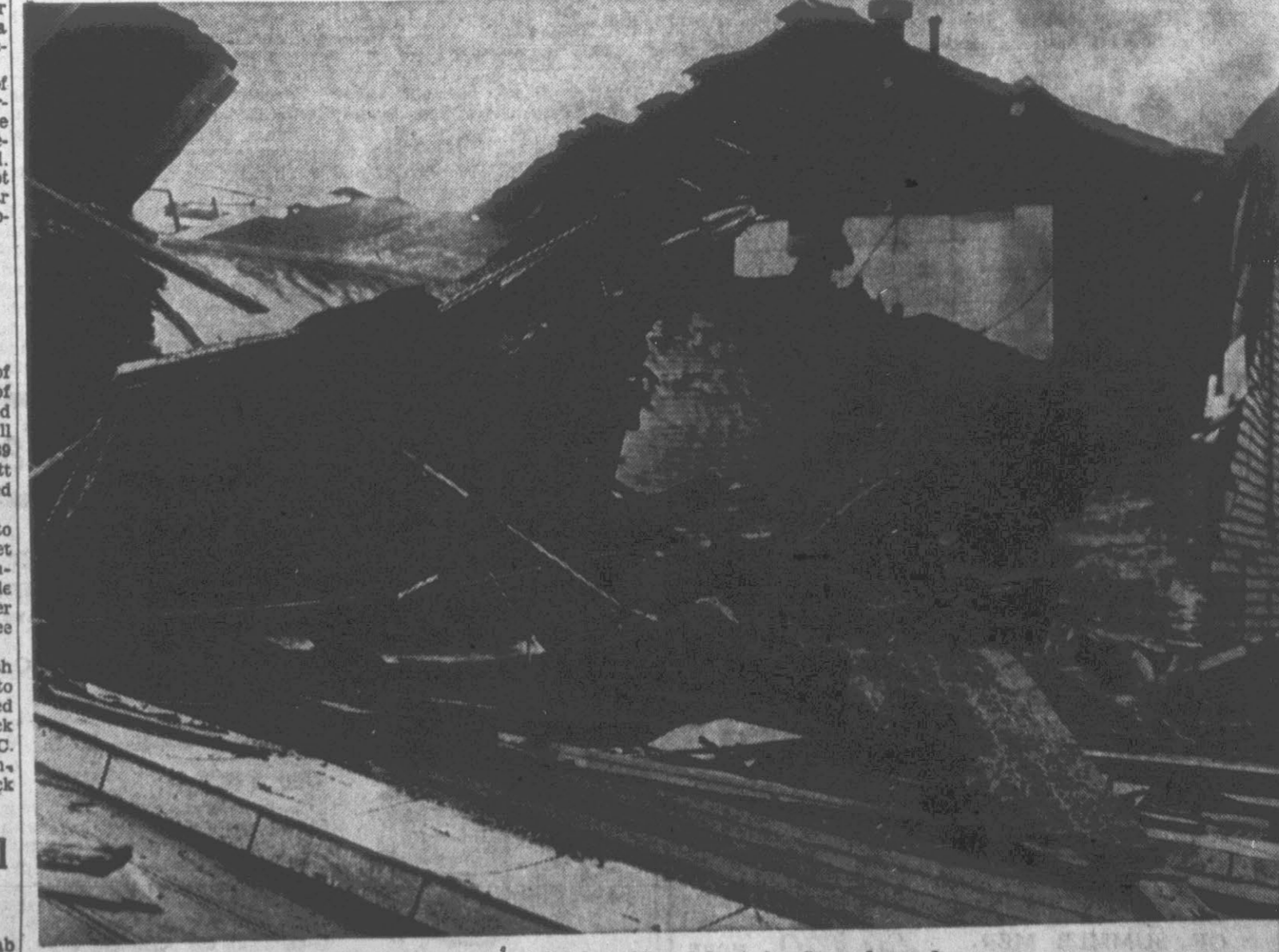
REMAINS . . . of the Plaza Theater which collapsed early Saturday afternoon.
