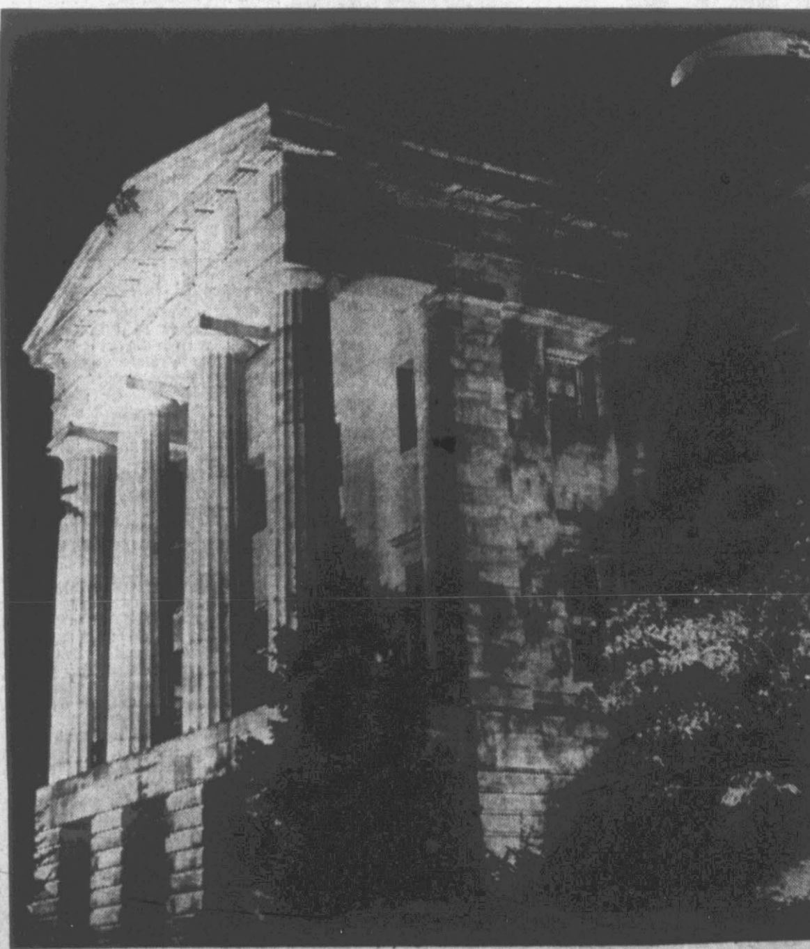
121-YEAR-OLD LANDMARK—North Carolina's State Capitol, with its majestic columns and entablature dramatized by floodlights, displays a classic blend of Grecian Doric and Roman Gothic architecture. Scotland's David Paton was the building's architect, designer and builder in the decade of the 1830s. The cornerstone was laid on July 4, 1833, for the entire tax that cost Tar Heels $531,674.46 over the 10-year period during a time when the entire tax structure for all State purposes totaled less than $100,000 per fiscal period. Copied from such immortal ancient Greek structures as the Parthenon, the Temple of Erechtheus and Lanthorn of Demosthenes, the classic masonry structure's night image was recently captured by Reflector staff photographer Stuart Savage
