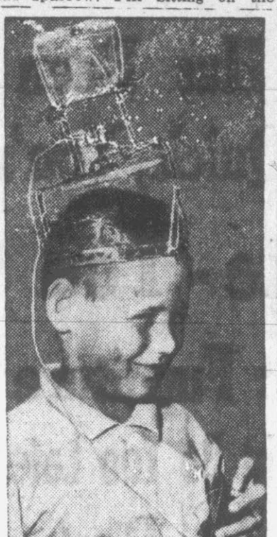
COOL TOP —Martin Ullman, 9, assembled a battery-powered motor, dry ice in container and a tiny fan into a heady cooler for the rising temperature at Miles City, Mont. screen.
