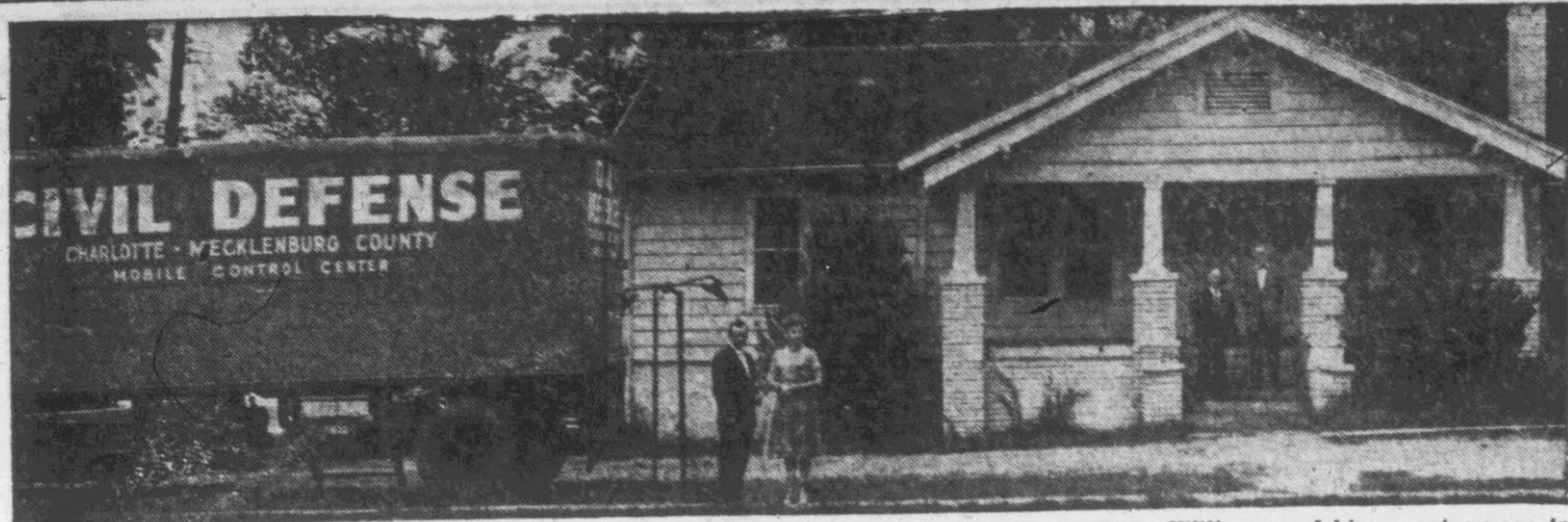
TANGIBLE PROGRESS in civil defense in Charlotte-Mecklenburg County, N. C., can be measured by the moving of its office from the trailer to the house, made possible by a new Federal cost-sharing program for State and local CD personnel and administrative expenses.
