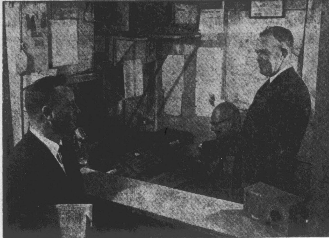
COMMUNICATIONS CENTER at Wadesboro, N. C., combines a round-the-clock civil defense nerve center with a unified radio service for local police, fire and sheriff's departments. Used for this dual purpose, the equipment is kept in top-notch condition at all times to meet emergencies. At the radio is Walde J. Stroud, one of three operators hired by the local CD unit under a program
