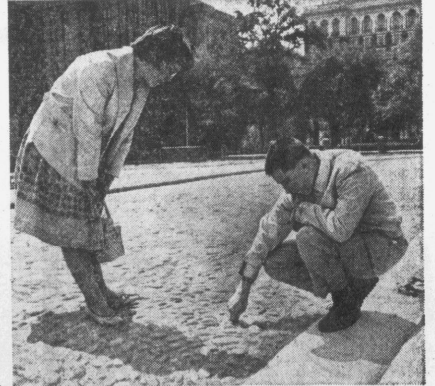
Patricia and James Lomako look closely at pebbled reconstruction of Library Street that runs from Independence Square to Carpenters' Hall in park.
