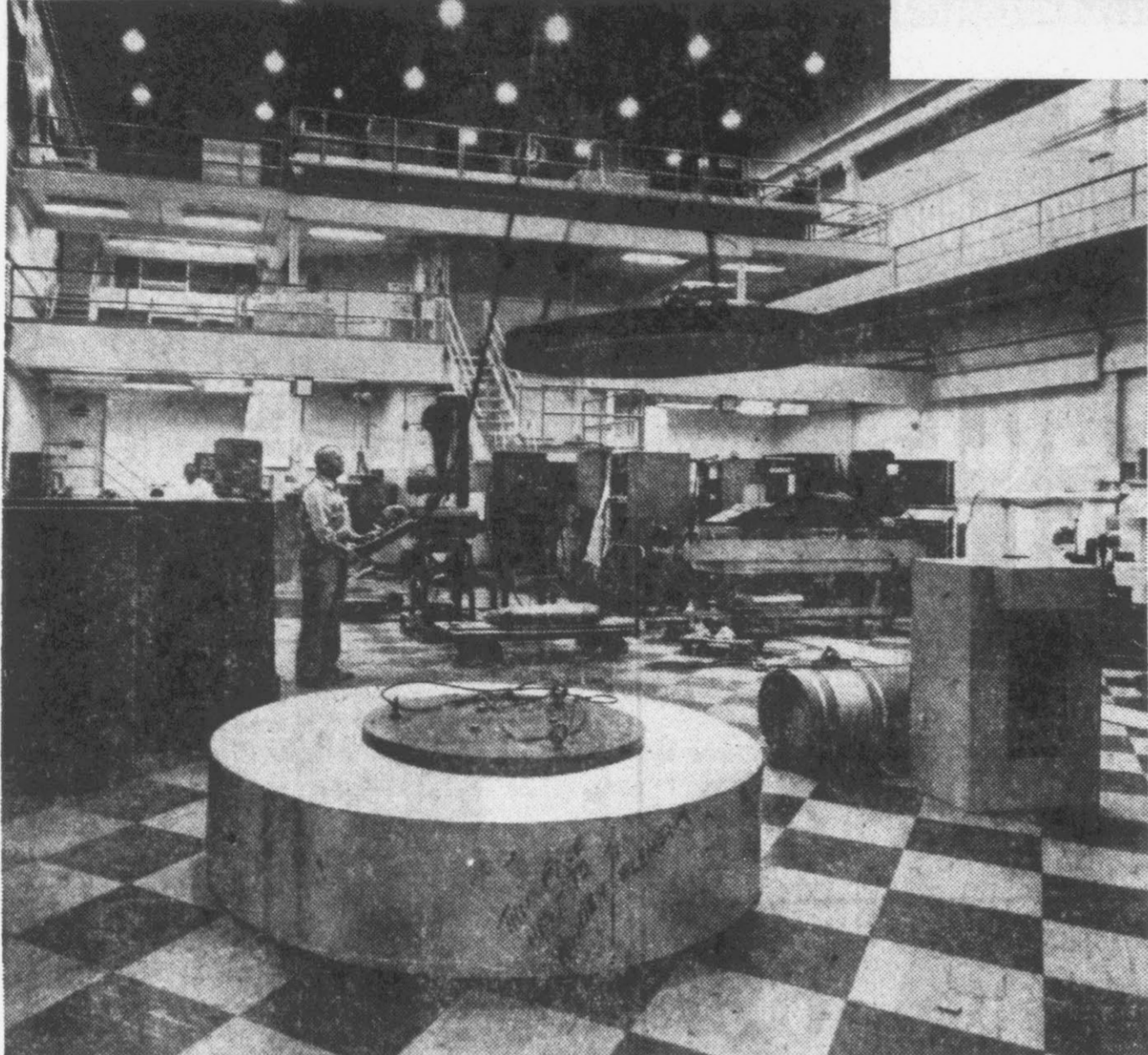
Experimental area of the Laboratory's nuclear reactor research facility. At far end of area is the reactor shield which contains beam ports. These are openings through which neutrons can pass for experimental purposes.
