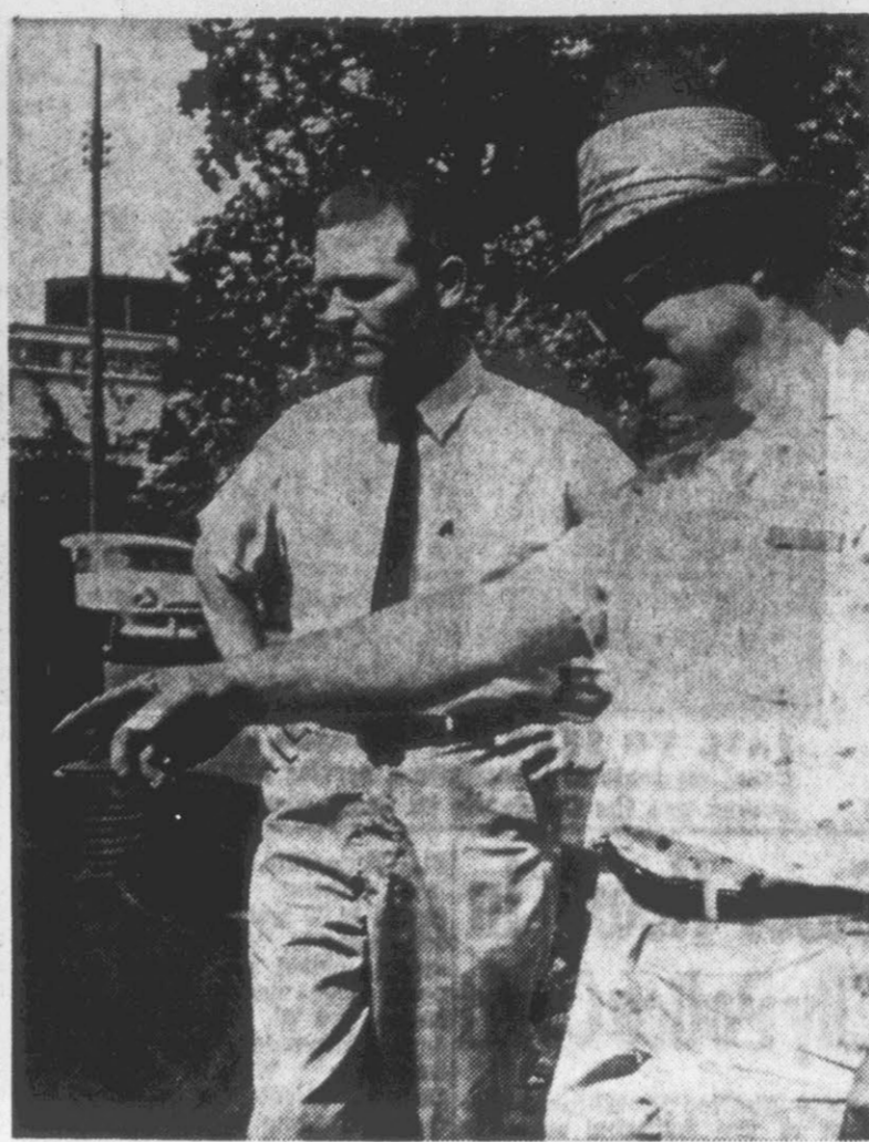
VIEWING CONSTRUCTION . . . work for improvements to city hall.
