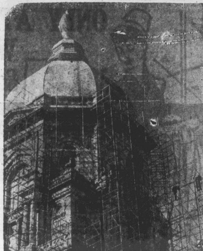
NEW COVER —Scaffolding is set around the Golden Dome at the University of Notre Dame prior to replacing the dome's sheet metal base and covering it with gold leaf.
