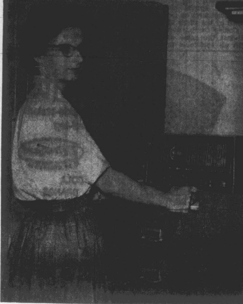
BASE STATION . . . for two-way radio system for the Department of Utilities and the Department of Public Works will be located in the Ayden Town Hall. Mrs. Peggy Bright illustrates the way the station will operate, with a microphone system. Installation of the system will provide quicker and more efficient service for customers, town officials stated. (Reflector Staff Photo)
