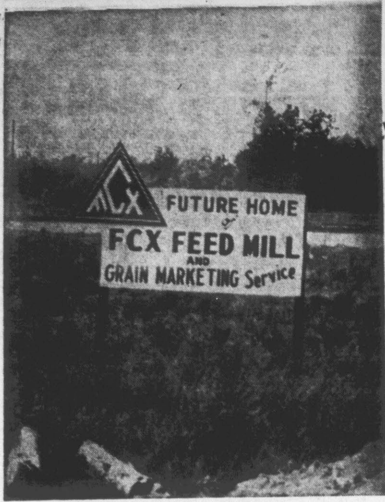
FARMVILLE GRAIN MILL SITE —Construction of a mammoth feed mill and grain storage facility by Farmers Cooperative Exchange, Inc., is expected to begin on this site within three weeks. Test boring operations to determine the type of foundations required for the FCX installation have recently been completed, according to company officials. Actual construction of the project—including facilities for storing some 300,000 bushels of grain—will require an estimated six months. The giant feed mill will be located on S. Fields St. in Farmville, just south of the Formica Flakeboard plant. (Reflector Staff Photo)
