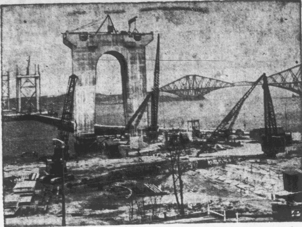
SPAN ACROSS FORTH —These towers will support the new bridge across the Firth of Forth near Queensferry, Scotland. When completed, the structure will be the longest suspension bridge in Europe. In the right background is the Forth railway bridge.
