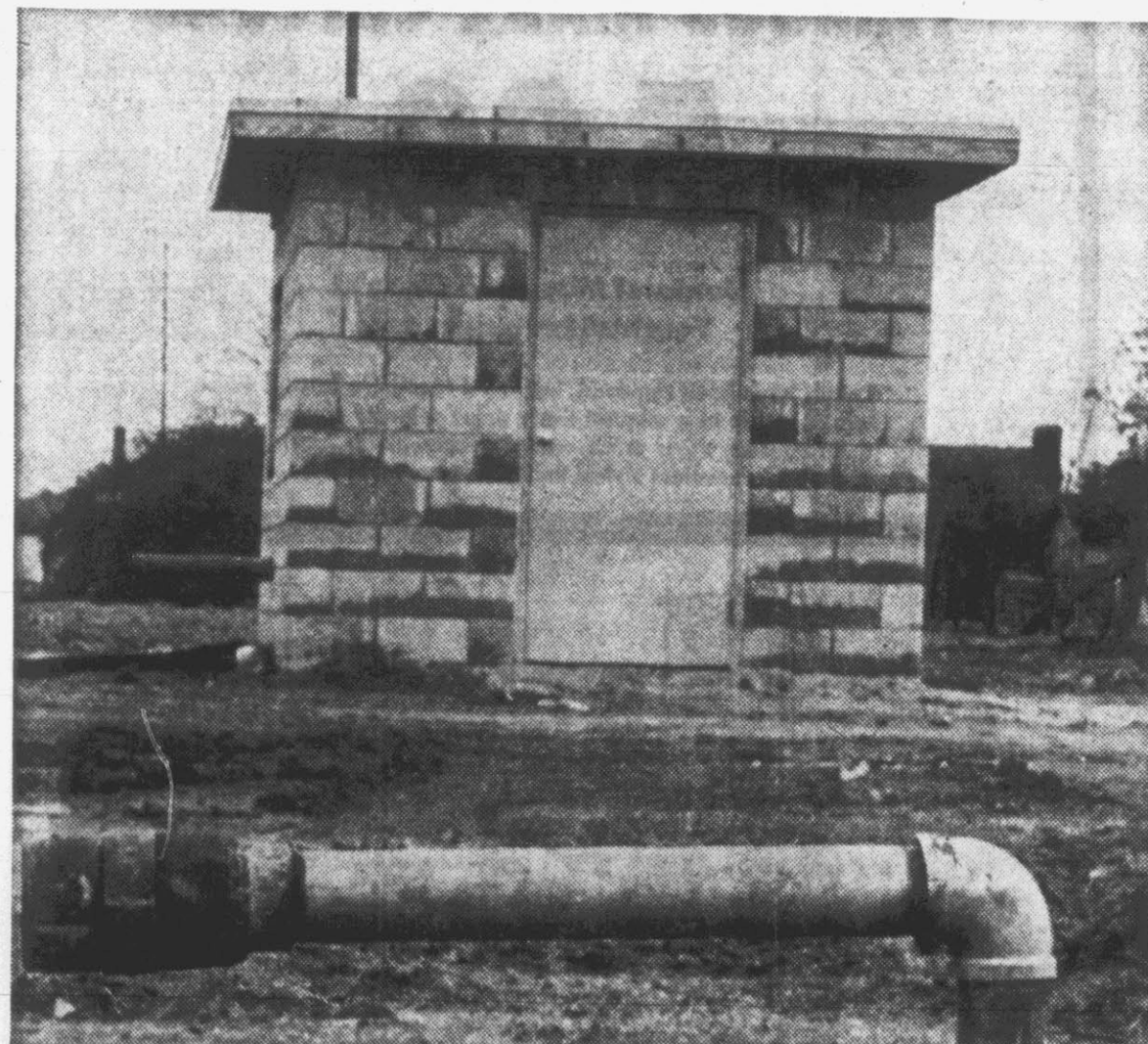
BETHEL'S NEW WELL AND PUMP HOUSE —A 400-foot well, with a capacity of 300 gallons of water per minute, was recently completed here. A pump house for the new pump was constructed at the well site which is located on the opposite side of town from the older wells. Completion of the project provides Bethel with three wells. (Reflector Photo by Stuart Savage)
