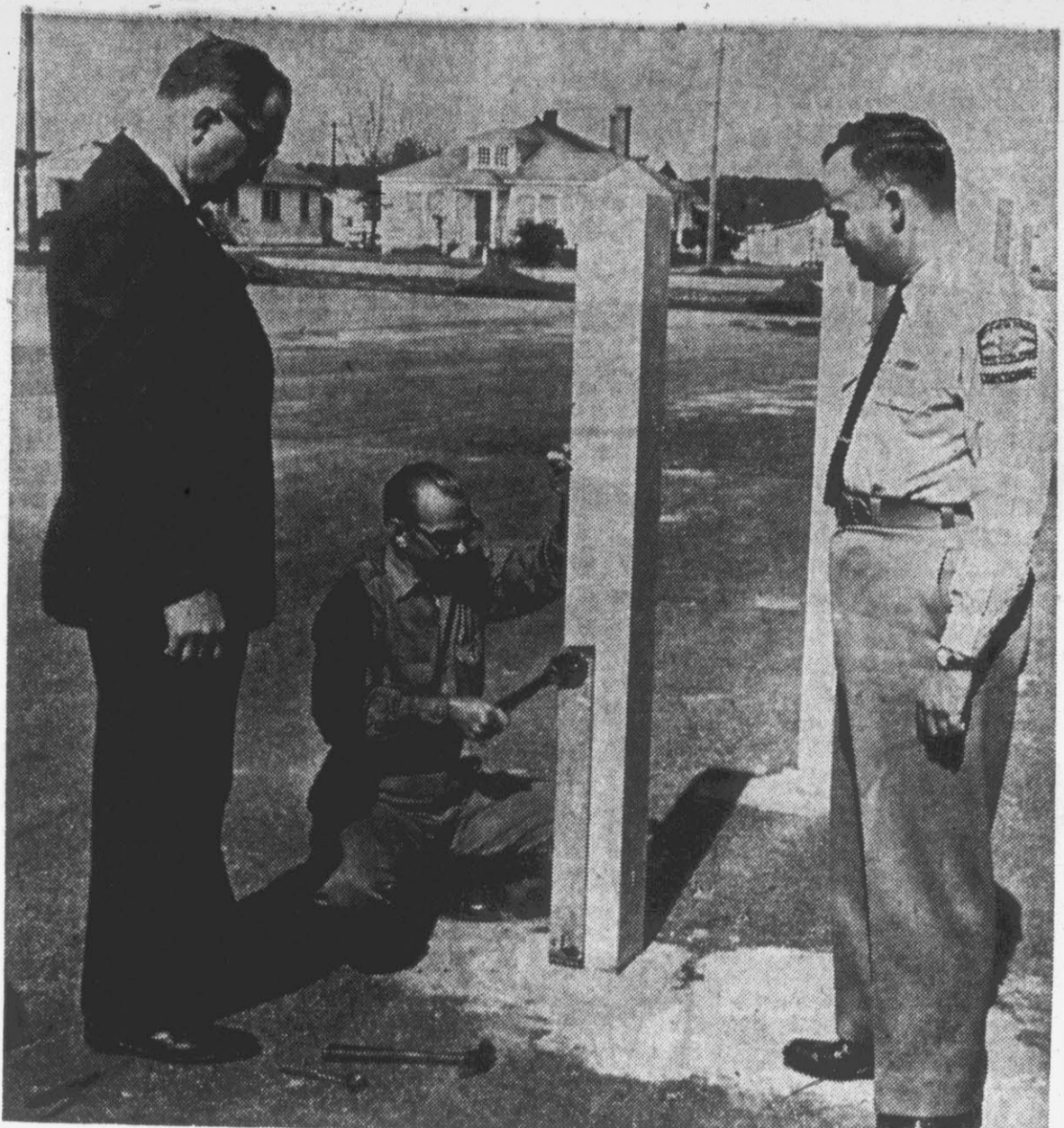
PRACTICE PARALLEL PARKING SPACE project, of Moose, looked over by Bynum and Grady. Now completed, the facility is available to use of general public.
