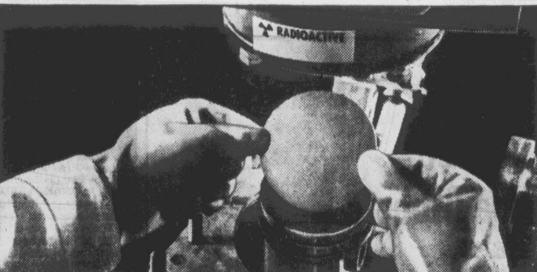
These gloved hands are placing a piece of sensitized film on a reactive piston. This produces what is known as a "radio autograph," from which Shell's scientists can study the nature of deposits.
