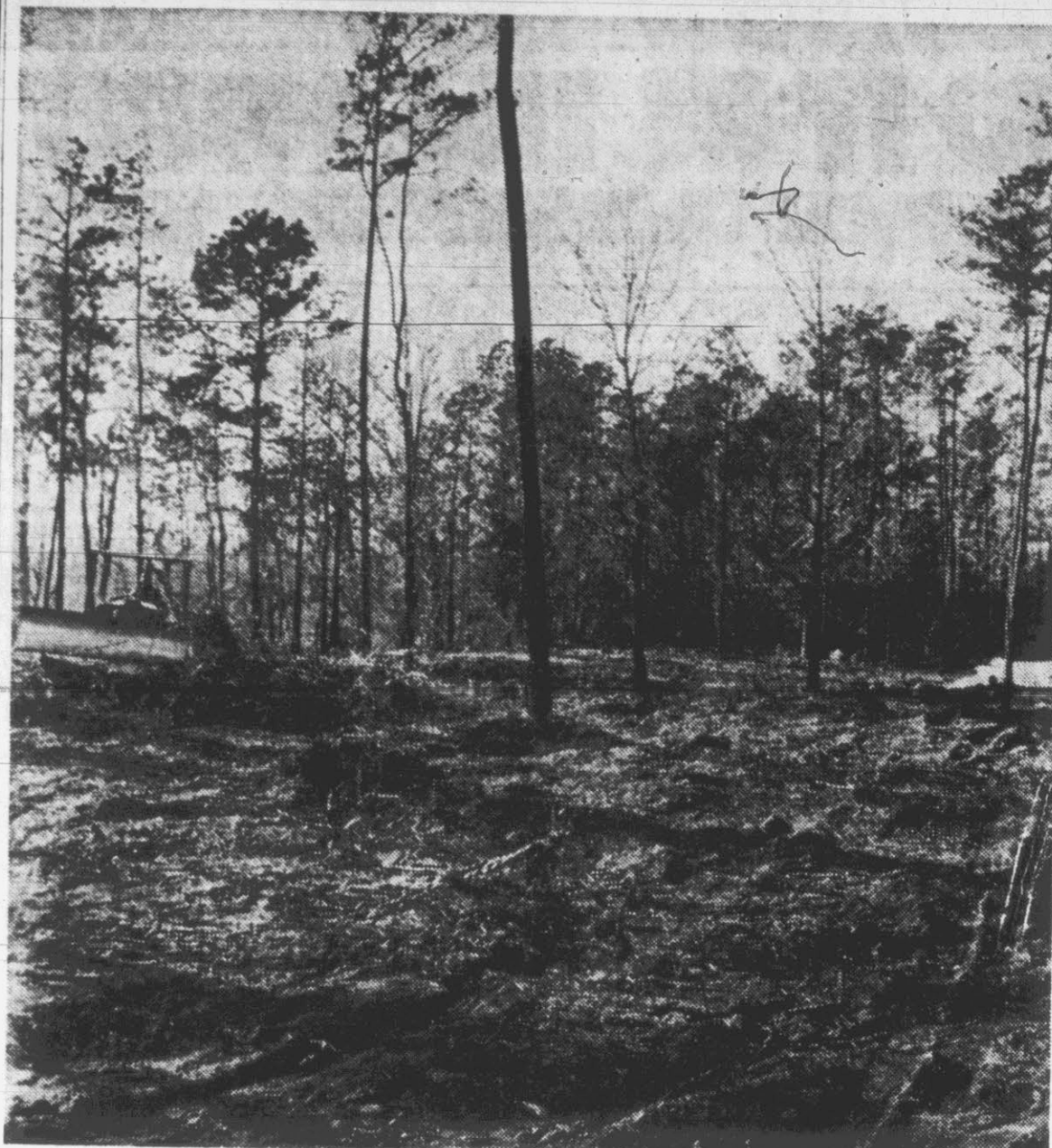
FOR FISHING ACCESS AREA —Contractors have been working for sometime clearing ground for construction of a fishing access area north of Greenville behind the Pitt-Greenville Airport. The three-acre plot is being developed by the Wildlife Resources Commission as a place for launching boats for recreational purposes in the area, and will include a paved launching ramp and a parking area. The project is scheduled to be completed within 60 days.
