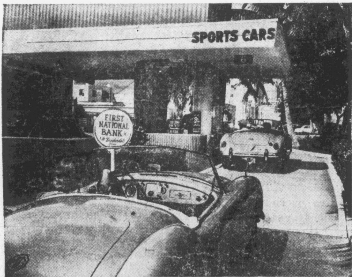
To accommodate sports car and small car drivers, this bank at Fort Lauderdale, Fla., built special elevated ramp at one of its drive-in windows.
