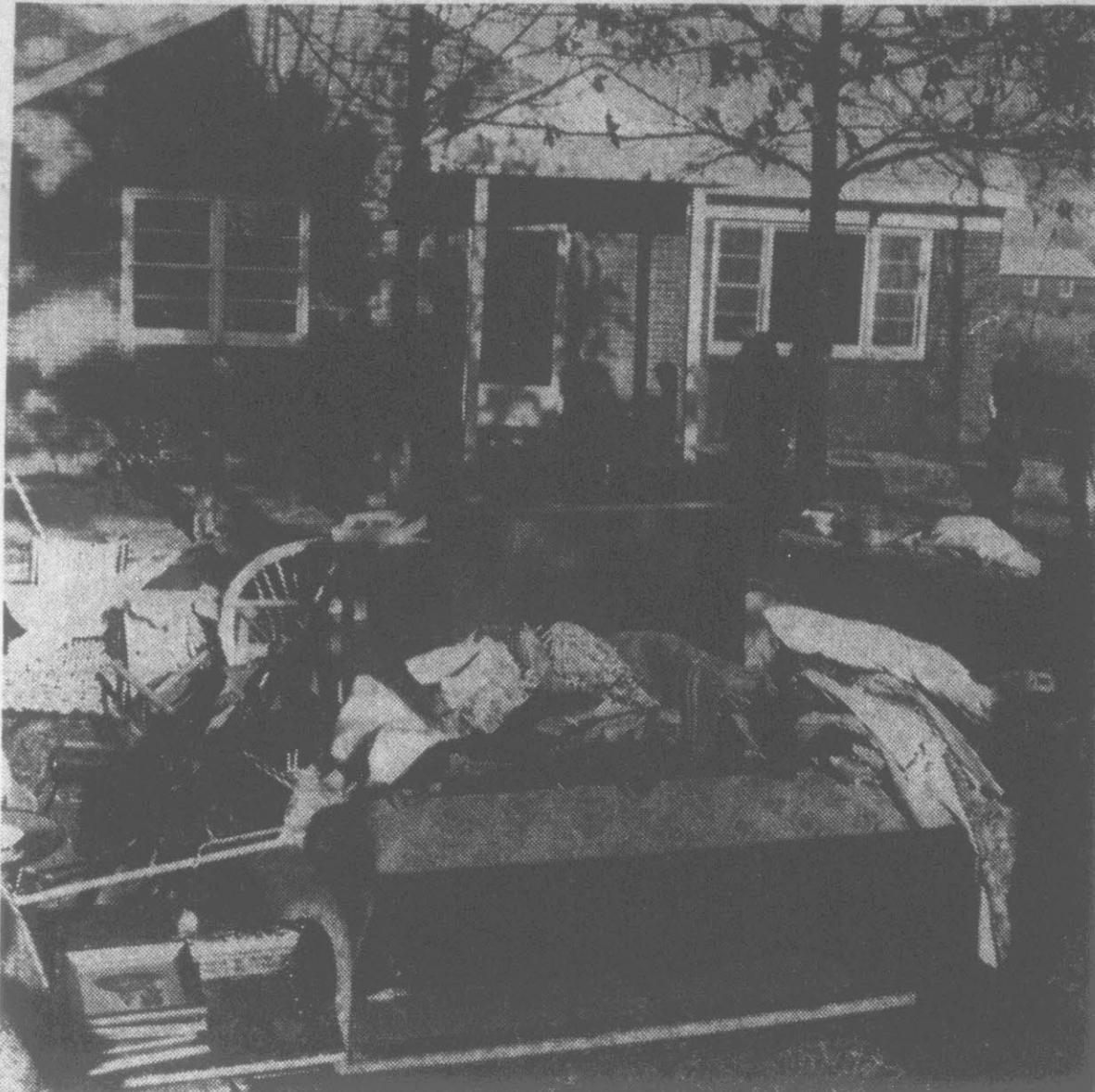
AT GRIFTON FIRE . . . furniture from the ground floor of the Edmondson home sits in a pile on the front lawn as firemen battle the blaze which gutted the second floor of the house. (Staff photo by Stuart Savage.)
