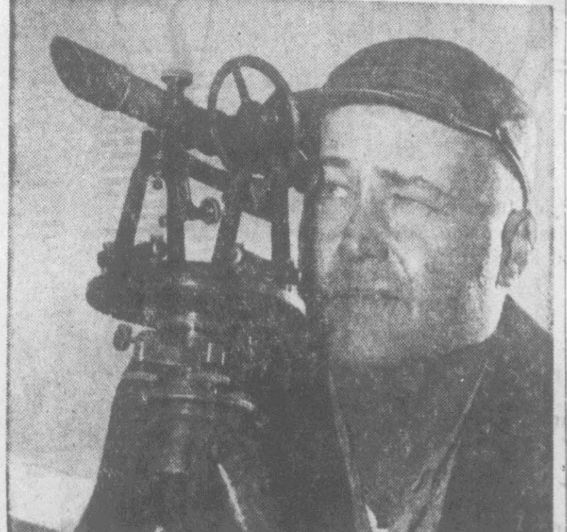
POWER LINE CONSTRUCTION . . . G. R. Spencer, construction foreman, charts course of a 70-mile, 110,000 volt line to serve Dupont and Voice of America Shermidine site.
