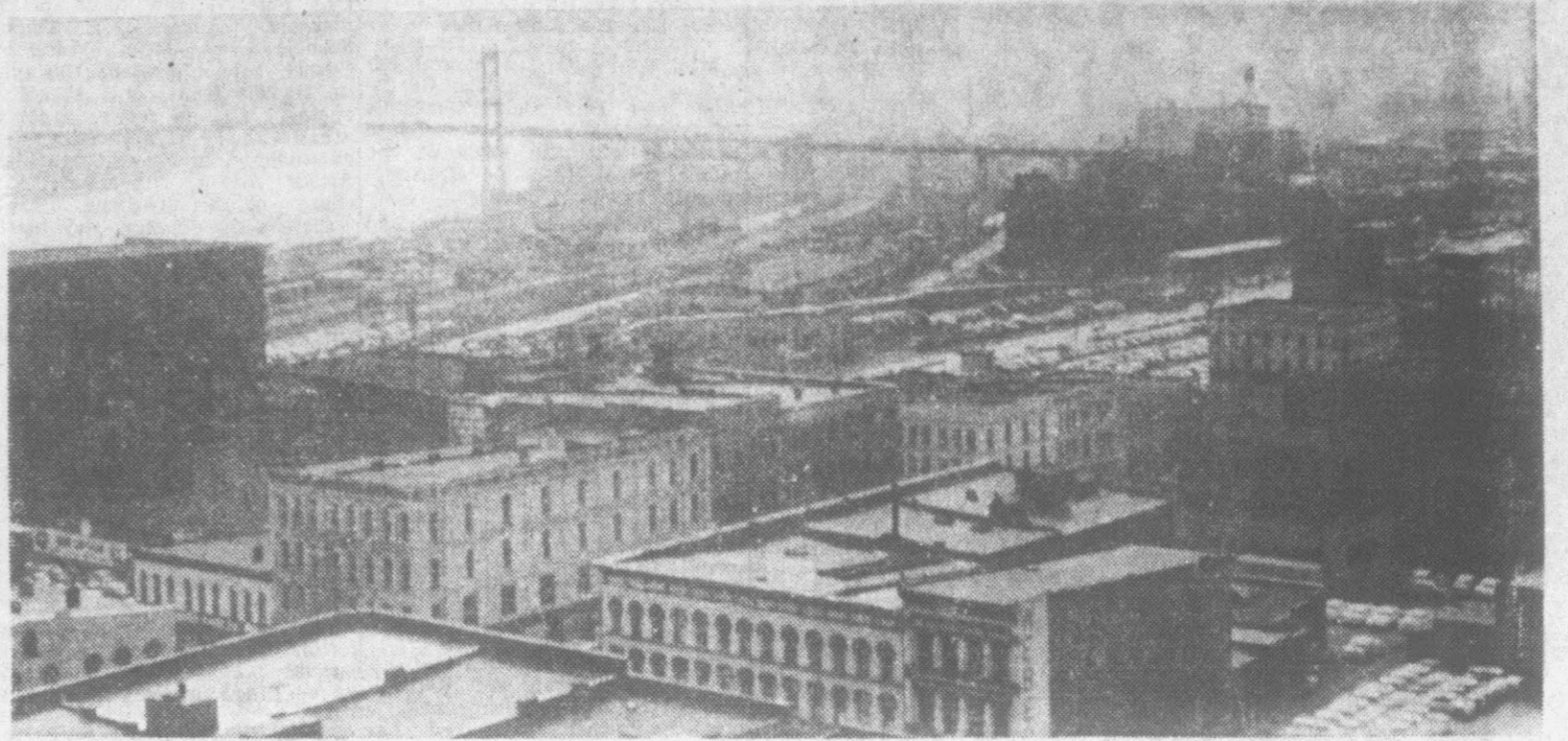
A MAJESTIC BRIDGE . . . spans Toledo's Maumee River.
