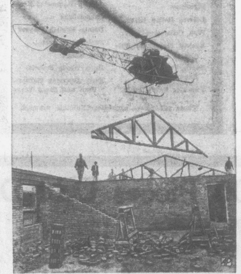
AERIAL FIT—Helicopter lowers gable frame into position on house in Denmark. Heavy rain made ground too soft to use a crane so a "copter" was pressed into service.
