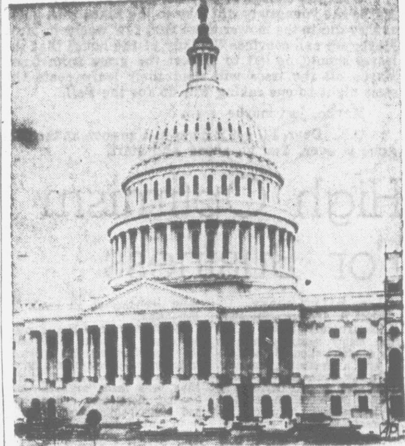
NEW LOOK — With the multi-million dollar improvement project almost completed, the east front of the Capitol in Washington, D. C. looked like this Oct. 8 — scaffolding removed and the dome glistening with new paint. Front of central portion was brought forward approximately 32 feet and all weakened structural materials were replaced or strengthened. Inauguration of new president will be held here in January, 1961. (AP Wirephoto)
