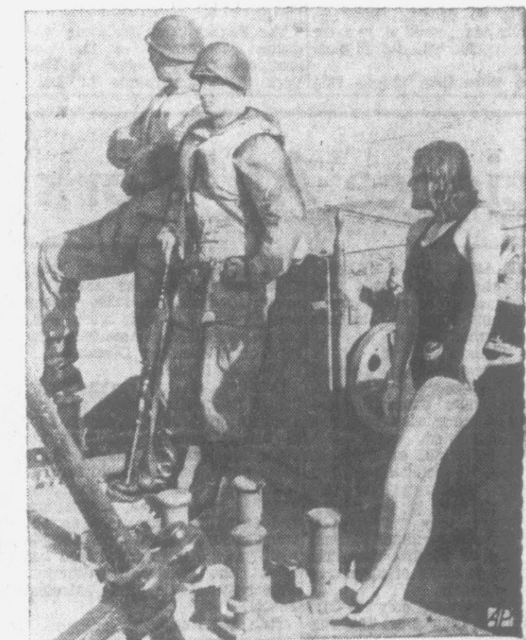
CIVILIAN AIDE—A female life guard is on duty with soldiers during building of pontoon bridge over Rhine at Duesseldorf during West German army maneuvers.
