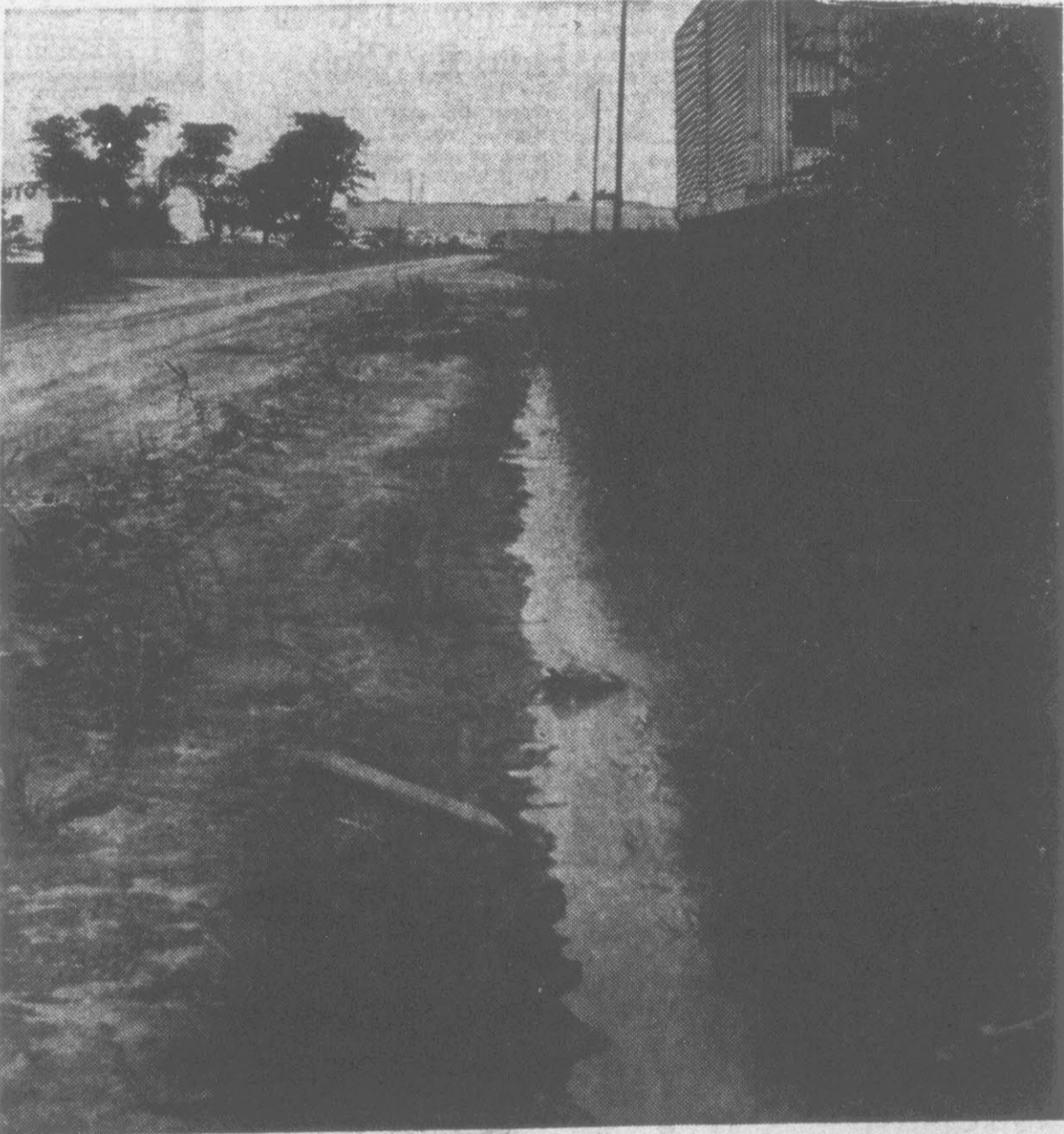
EVENTUAL PAVING FOR MOST DIRT STREETS . . . with revolving fund which bond issue established.
