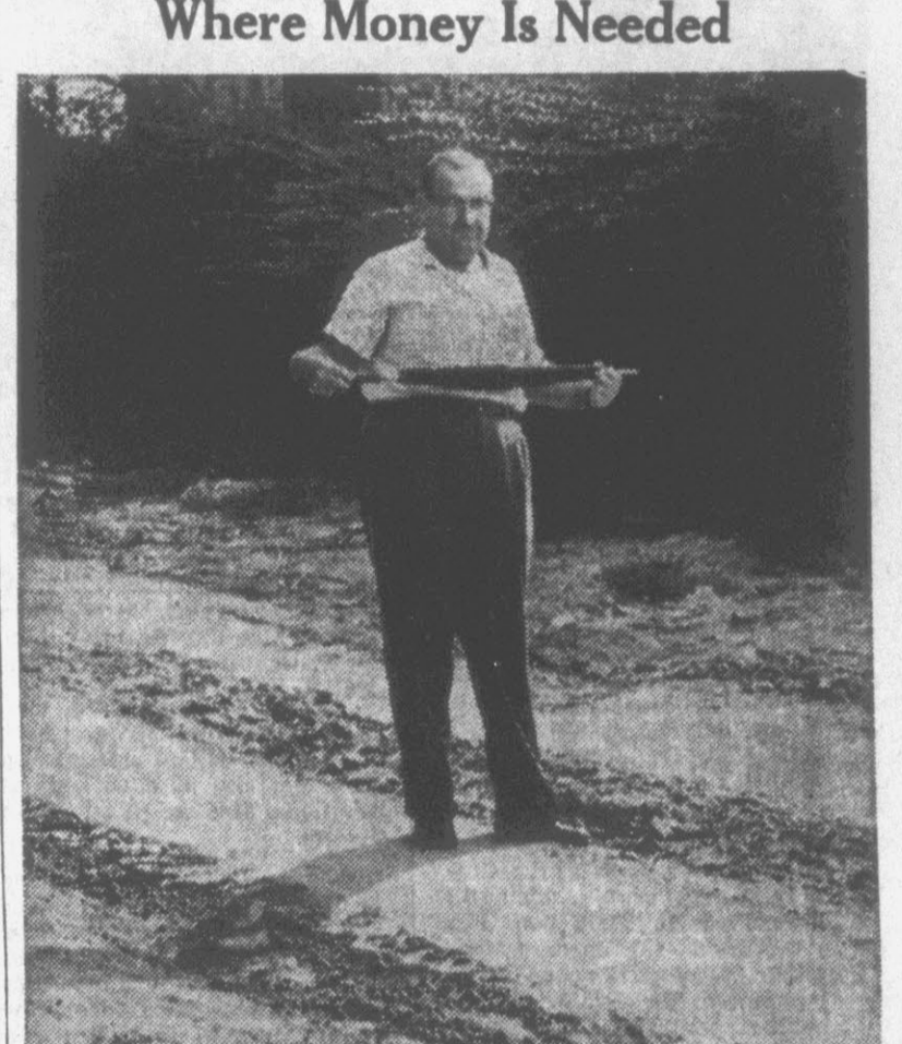
STREET PROBLEMS . . . City Manager Bloxam indicates street erosion with umbrella.
