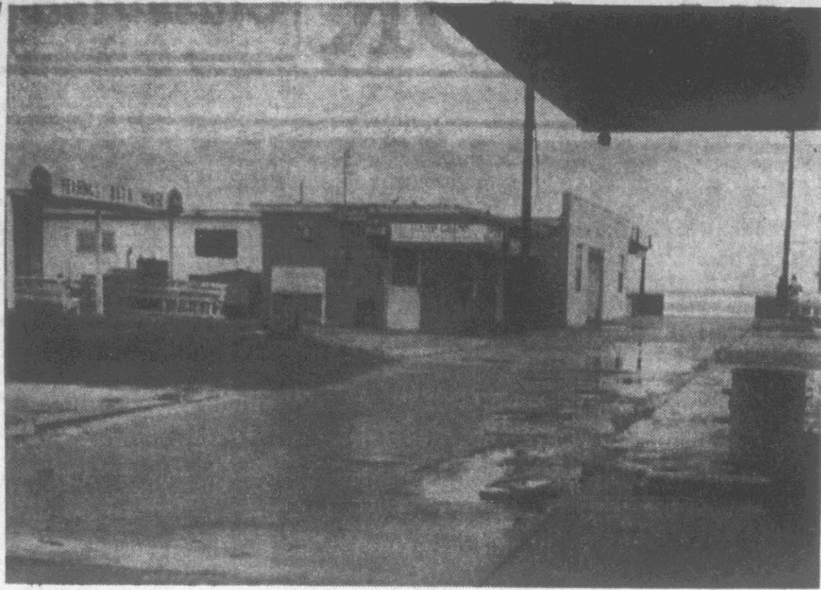
ONE OF THE MAIN ENTRANCES . . . to Atlantic Beach looked like this early Sunday afternoon while Hurricane Donna was still many miles from the North Carolina coast.
