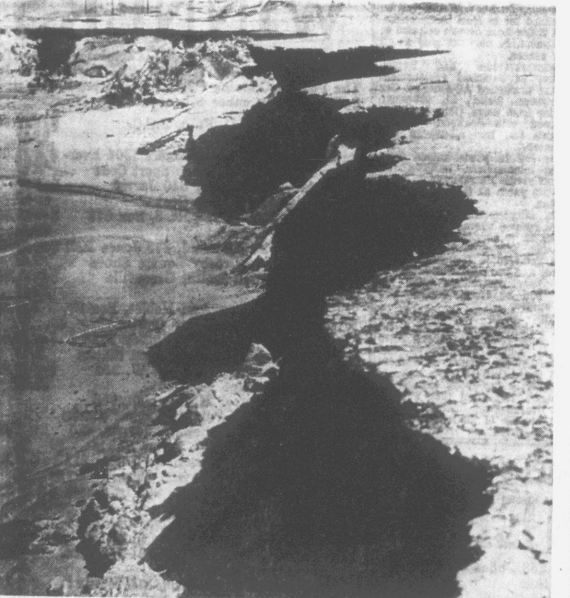
THE EMERALD ISLE ROAD . . . between Salter Path and Emerald Isle was made impassable when the ocean washed this huge section of asphalt away, leaving nothing but a gaping hole. (Photo by Roy Hardee)
