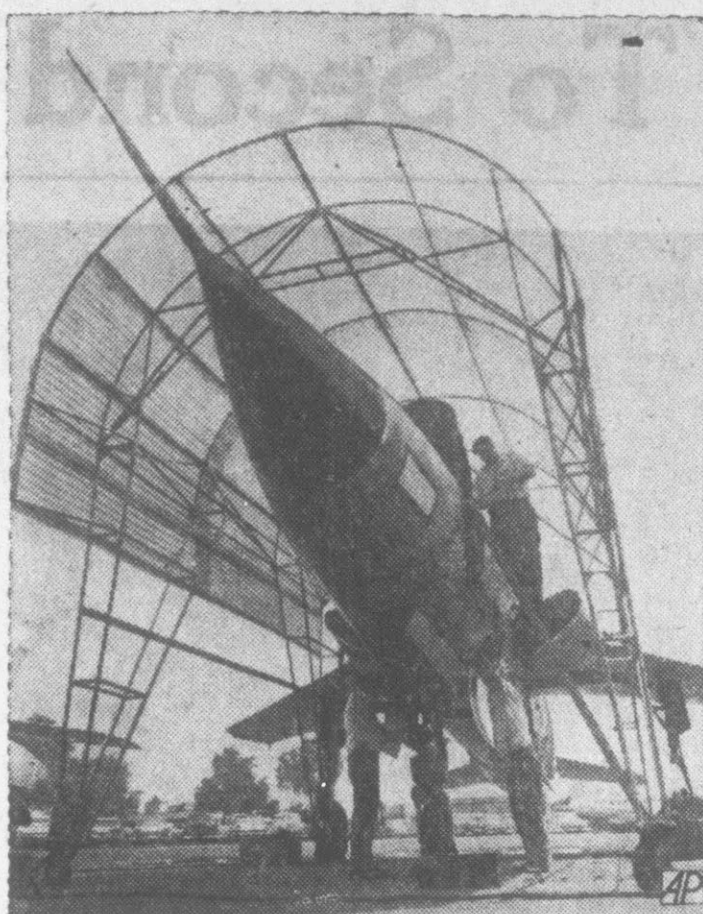
WORK COVER —A fiber glass canopy provides all-weather protection for technicians installing electronic gear aboard a F-105D jet fighter-bomber at Farmingdale, N. Y.
