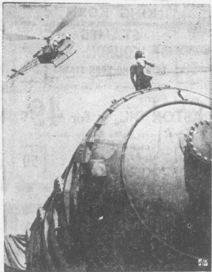
DUAL TASK — Man with walkie-talkie and a helicopter combine forces in intricate job of "bedding down" a 42-ton experimental space chamber at Farmingdale, N. Y., site.
