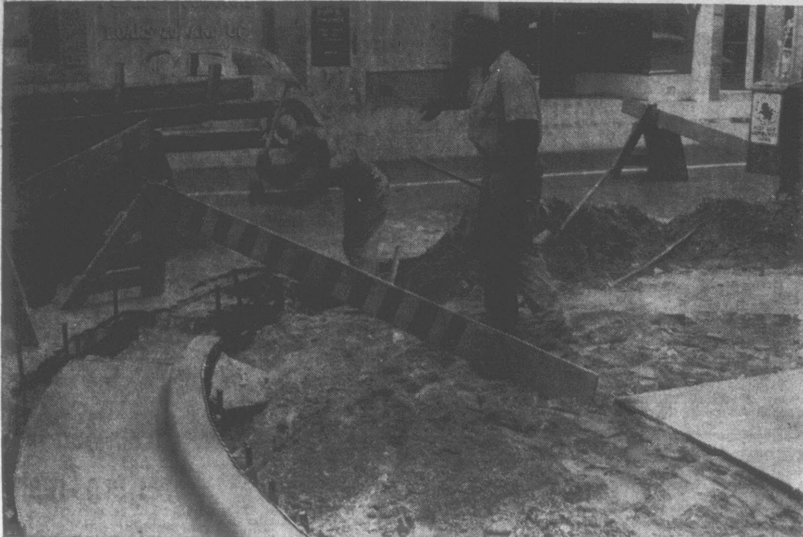
NEW CURBING—City crews are placing new curb and gutter around the turn in front of State Bank building and for a distance along Fifth St. City Manager Leonard Bloxam said the curb in front of the building had settled almost flush with the street so that water flooded the sidewalk during rains. Cars also ran on the sidewalk in making the turn, creating a pedestrian hazard, Bloxam said. The project will cost approximately $400. (Reflector Staff Photo)
