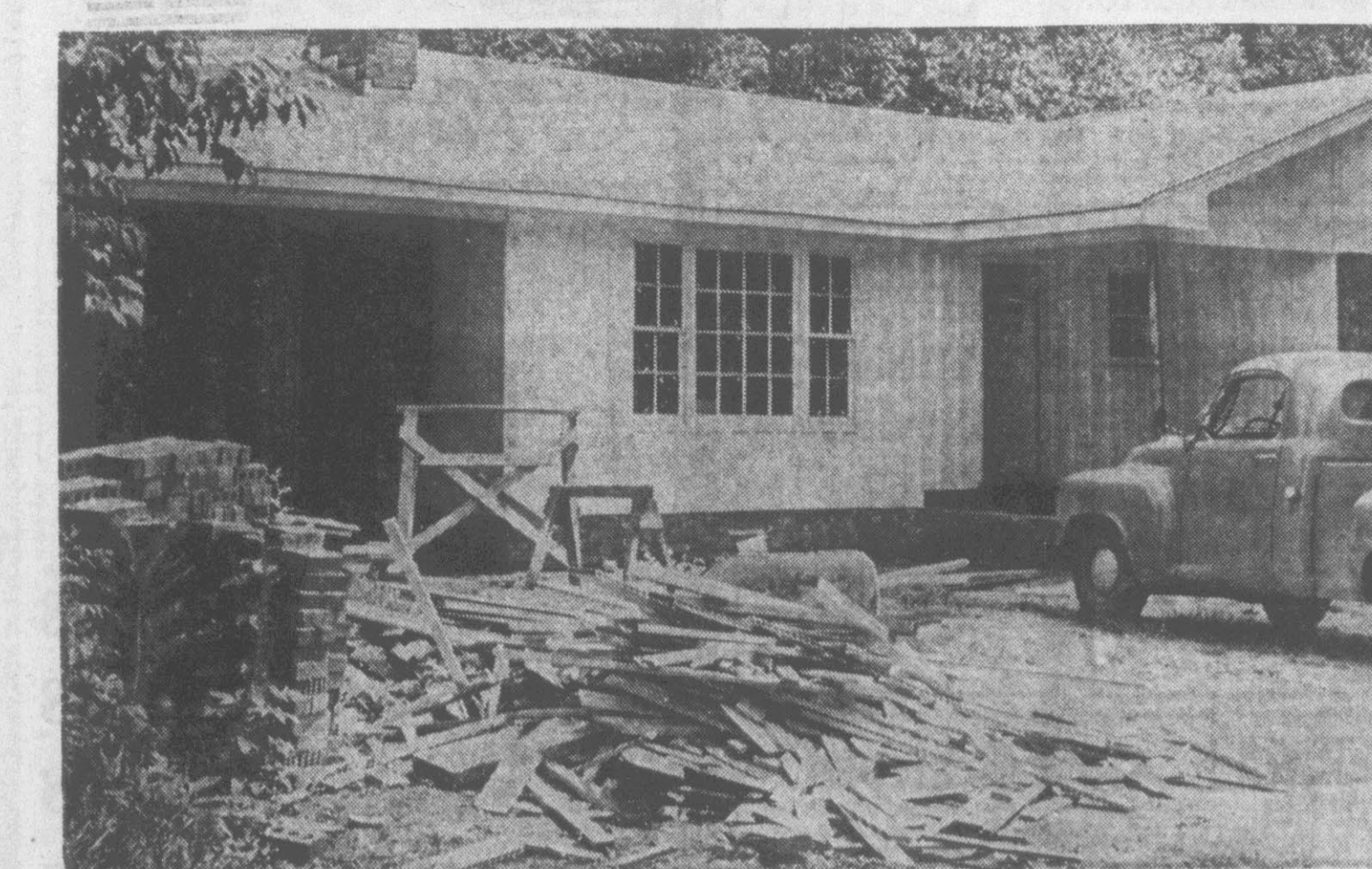
HOUSE BUILDING LEADS FIRST SIX MONTHS . . . dwelling construction amounts to $669,700.
