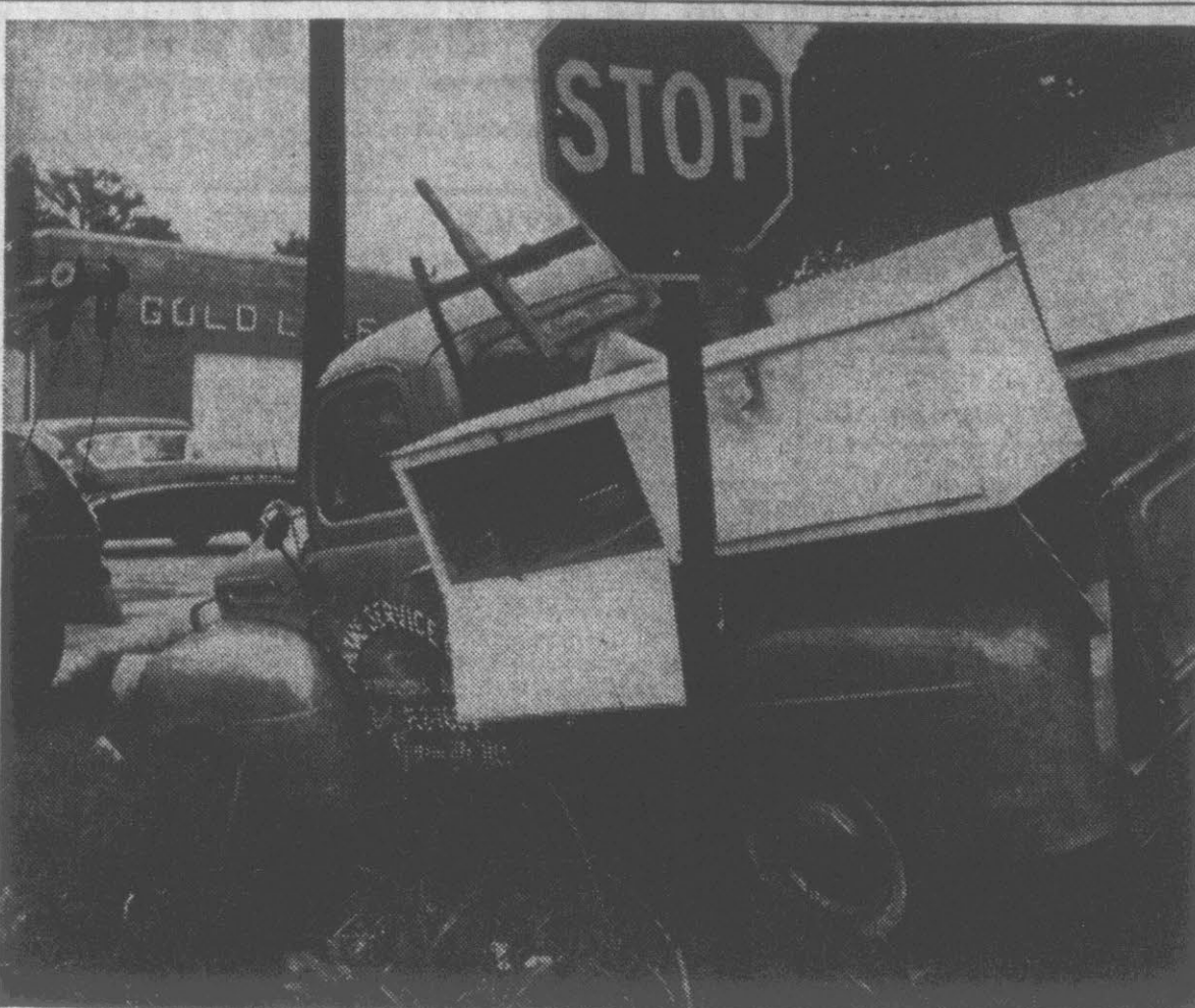
A NEAR MISS . . . is what this truck had yesterday. It stopped inches away from Charles Street, after its brakes failed and the driver pulled to the right and into the embankment in an effort to prevent a serious accident.
