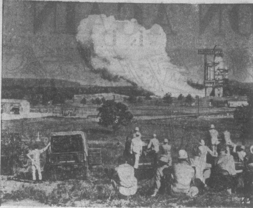
TESTING THE POWER —The eight engines of the giant Saturn rocket spew smoke in final static test of the current series at the Marshall Space Flight Center in Huntsville, Ala. In the 122-second test, the engines generated 1,300,000 pounds of thrust.
