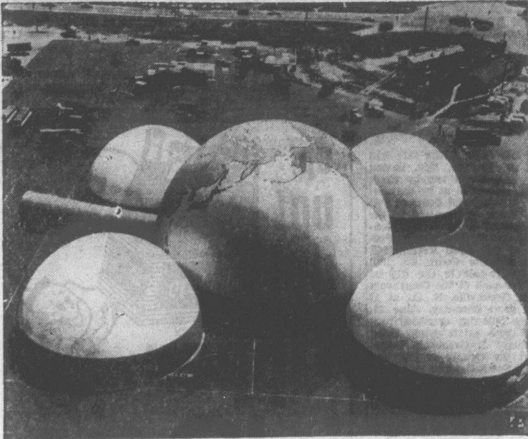
VILLA FOR MISSILES - These five plastic-roofed domes, the largest as tall as a nine-story building, are used for missile maintenance at Andrews Air Force Base in Maryland. The air-supported bubbles can withstand winds of hurricane force.
