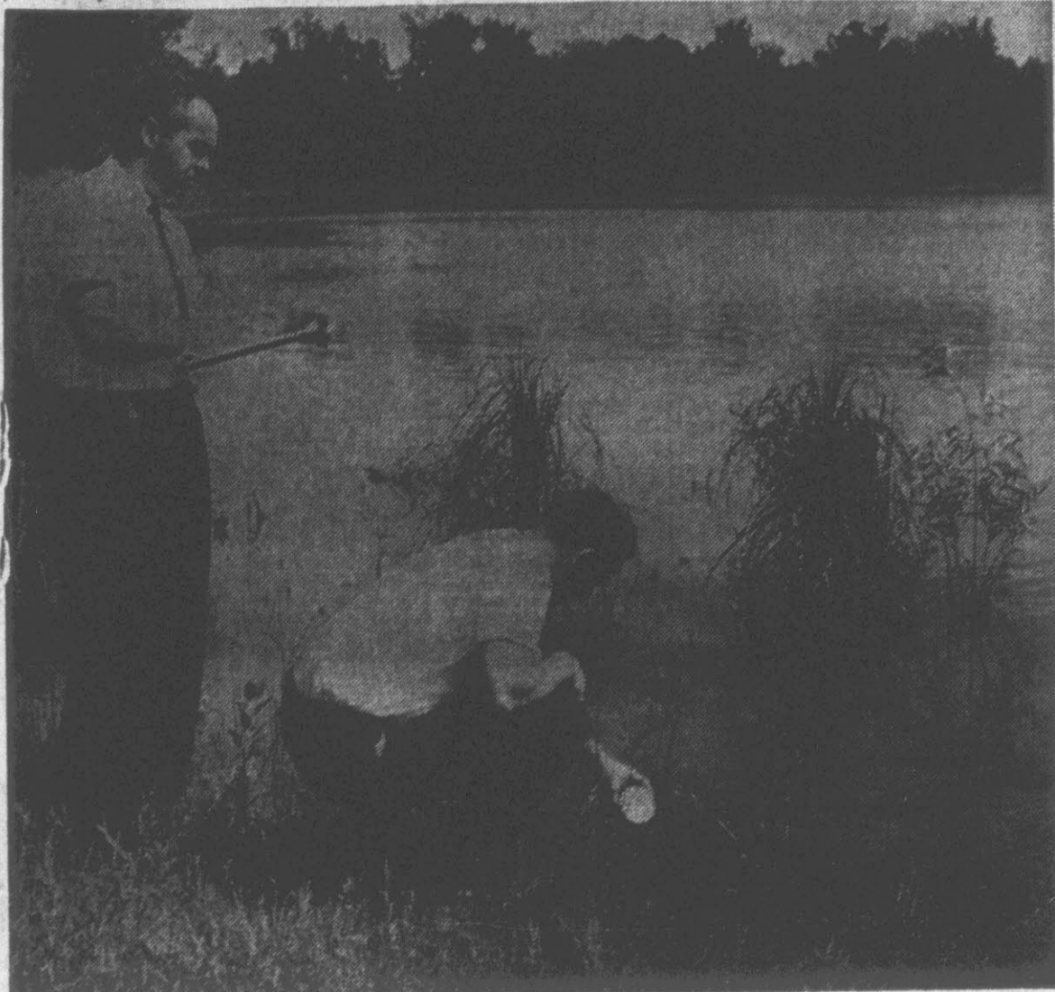
PITT POND CHECK . . . Kilpatrick (left) makes notations on possible mosquito hazards while Wood takes water sample to determine larva content.
