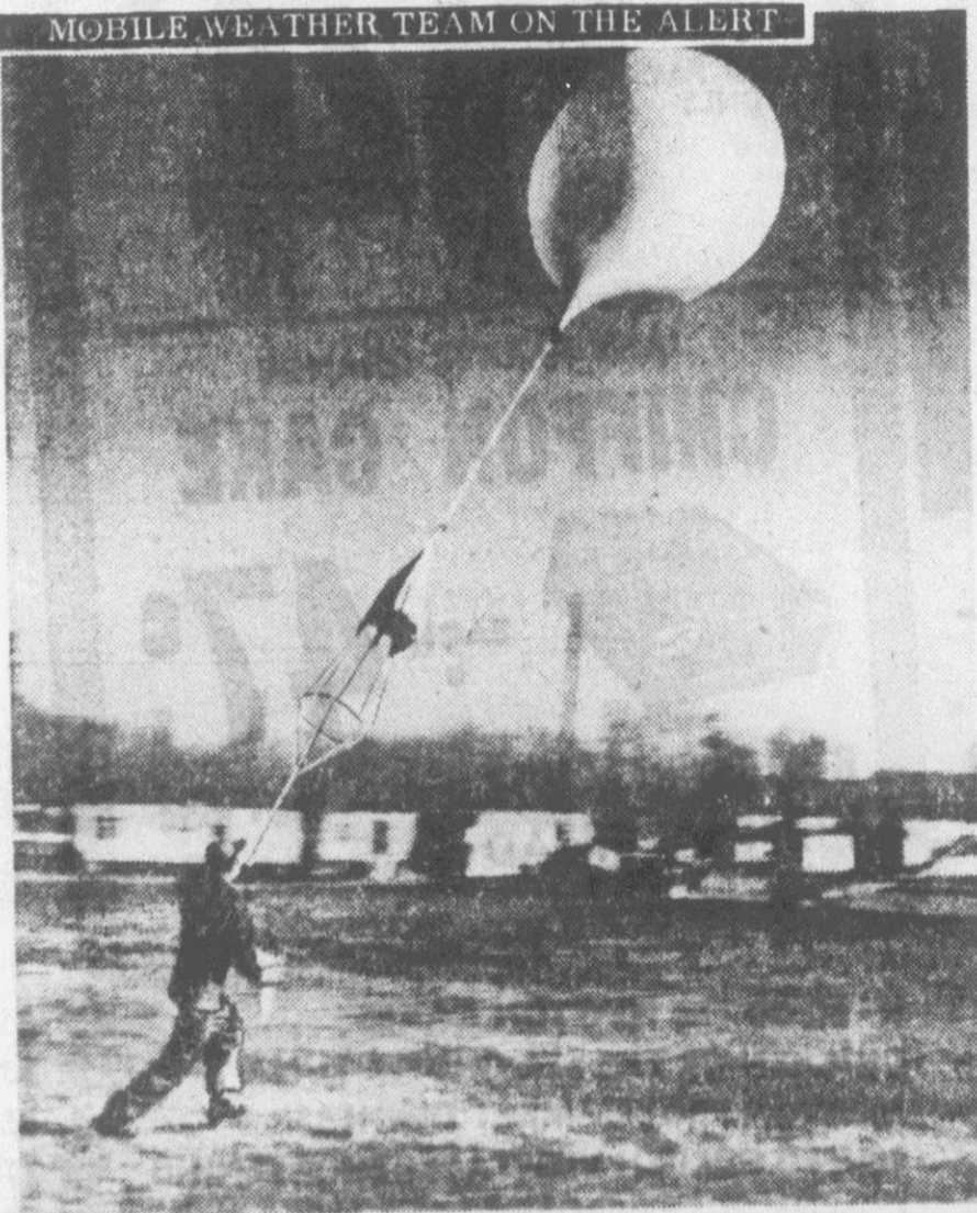
At Reese, Tex., where Air Force mobile team is on alert for twisters, Airman W.G. Workman releases balloon with radio equipment attached. Data on air conditions at various levels is signaled back to recorder on ground.
