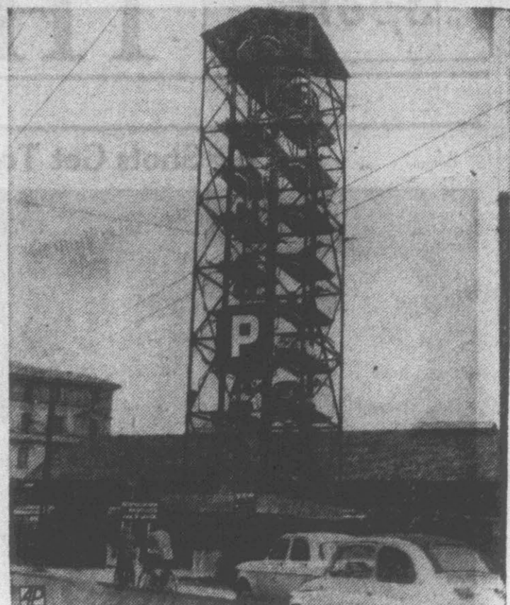
NO ROOM BELOW — This metal structure in Milan, Italy, is one solution to the parking problem. Cars driven onto elevated platform are stacked up in boxes.
