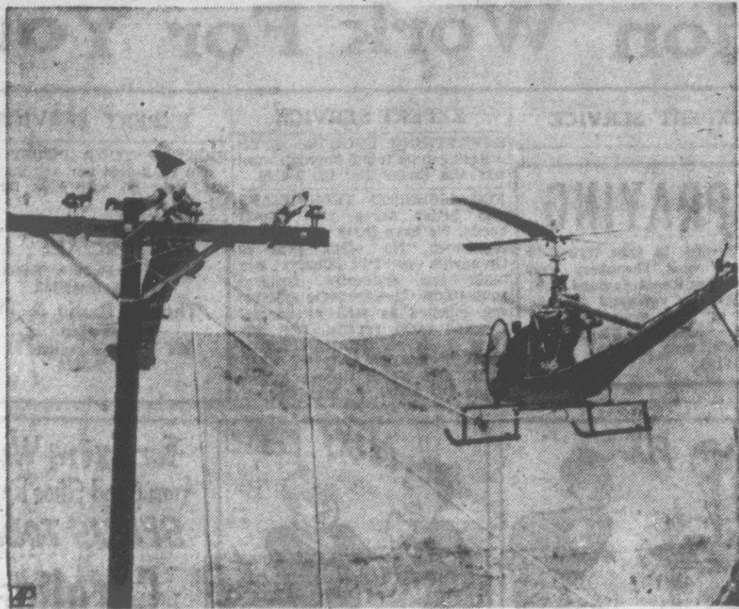
AN AERIAL ASSIST - Lineman guides power line through pulley over king pole as pilot Wes Lematta moves helicopter away after delivering the line at Rufus, Oregon. The 'copter also set poles in this first venture of its type in the Northwest.
