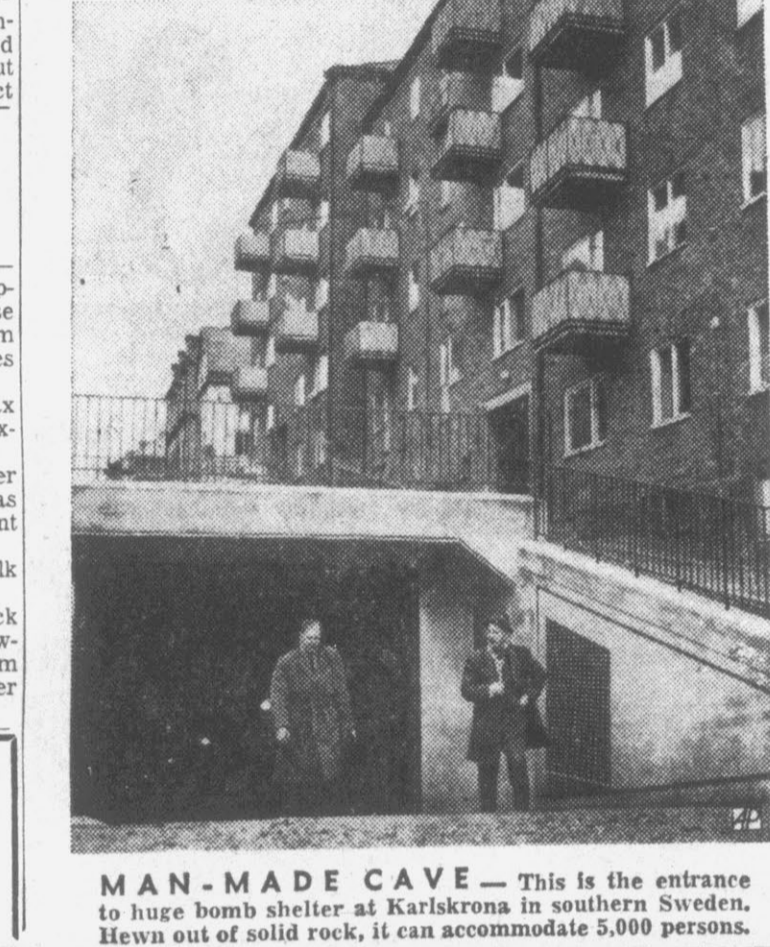
MAN-MADE CAVE— This is the entrance to huge bomb shelter at Karlskrona in southern Sweden. Hewn out of solid rock, it can accommodate 5,000 persons.
