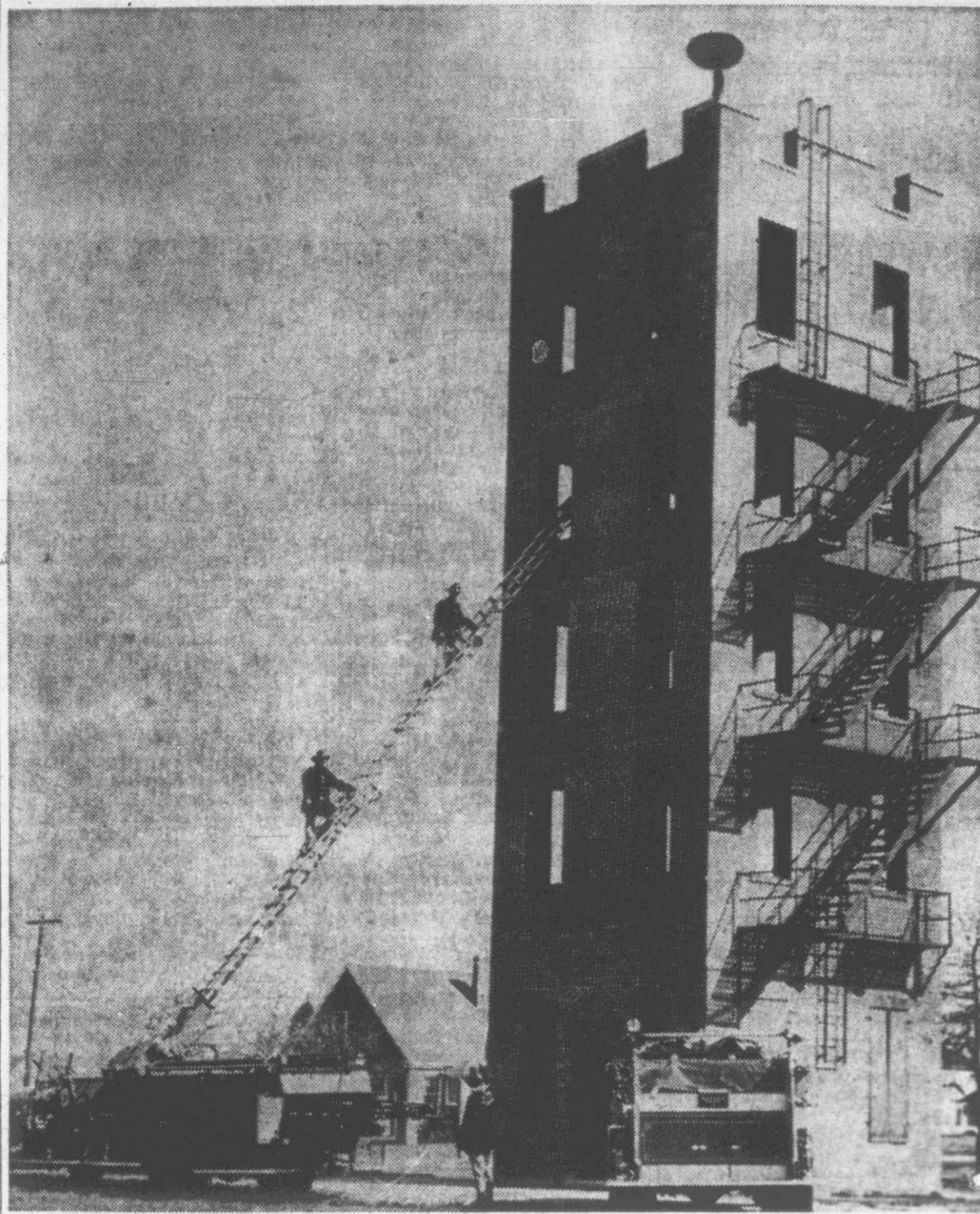
PROPOSED SMOKE HOUSE . . . to be supported financially by The Greenville Saddle Club with their Horse Show proceeds, will join above tower in further equipping the local fire-rescue training facilities.
