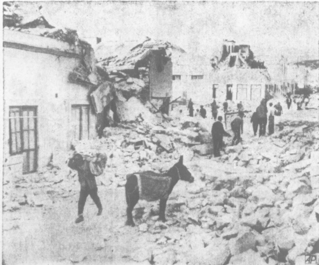
DEATH OF A CITY — Crushed by earthquakes and a tidal wave, the Moroccan city of Agadir is a heap of wrecked buildings and rubble. Survivors salvaged some possessions from homes before the city and its thousands of dead were abandoned.
