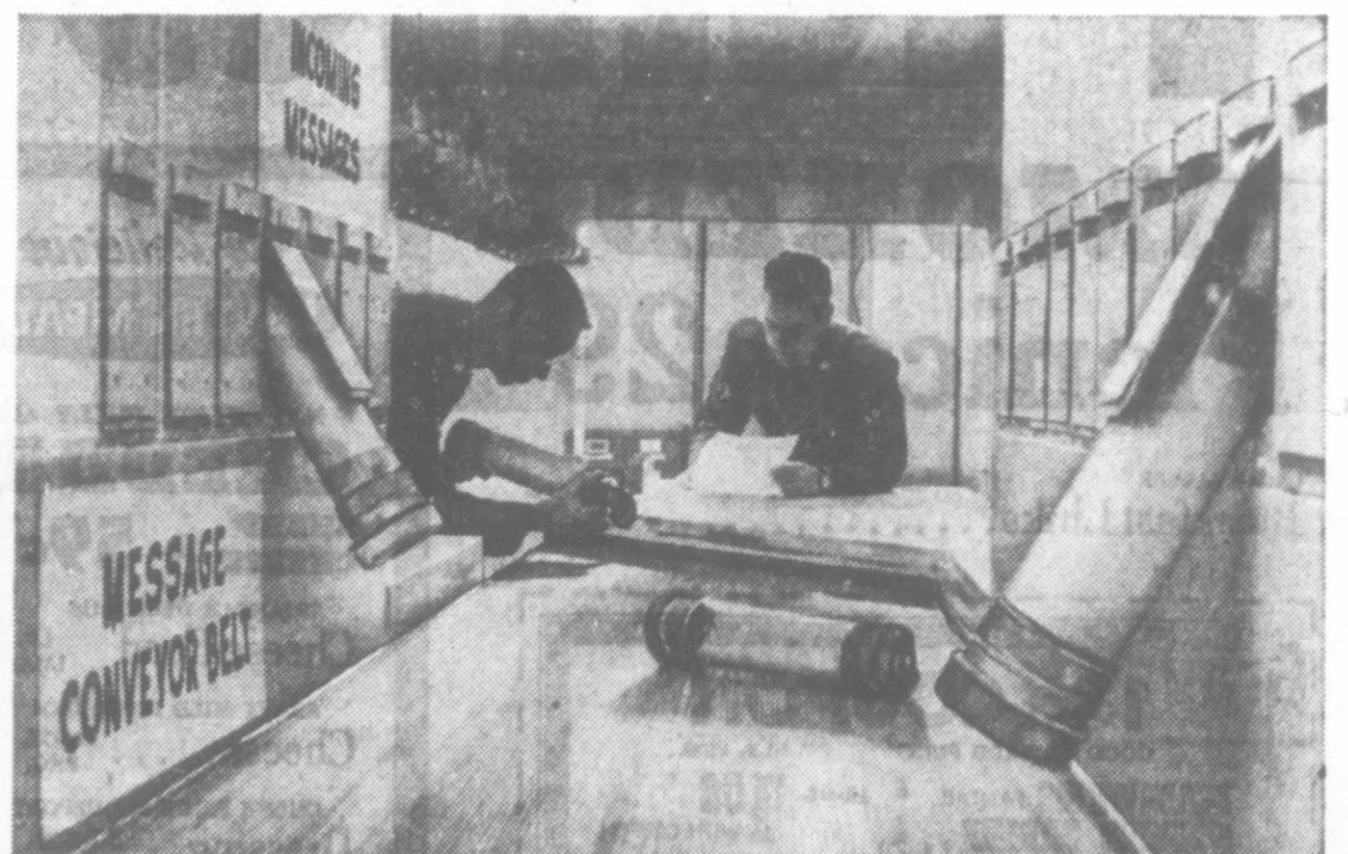
Message center where clerks take messages coming in from all parts of headquarters by pneumatic tube and distribute them for transmission, and vice versa.
