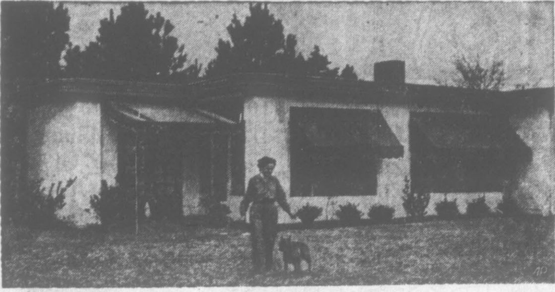
BUILT OF DIRT—Mrs. Lincoln Dowdy stands in front of the rammed-earth house she and her husband bought 12 years ago. The house has walls 18 inches thick.
