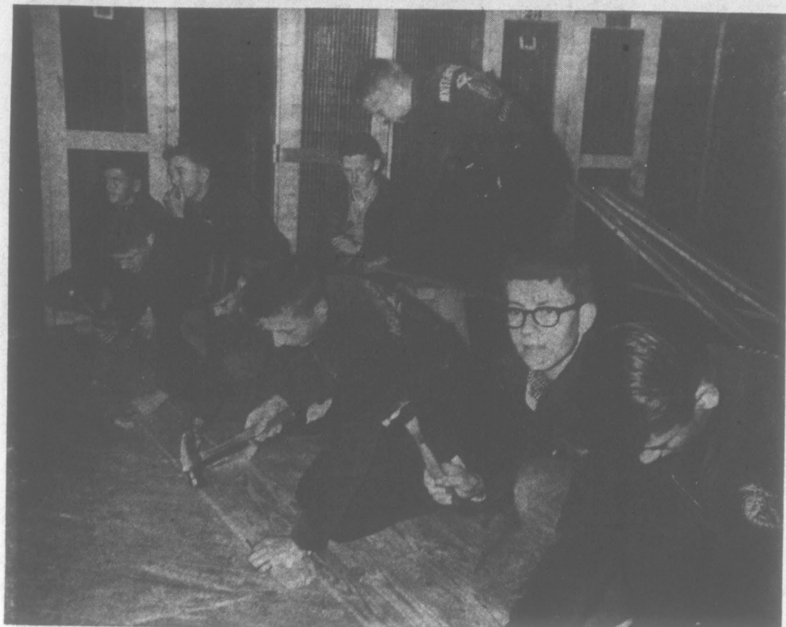
GRIMESLAND FFA MEMBERS MAKE BUILDING IMPROVEMENTS . . . boys, above, install flooring.
