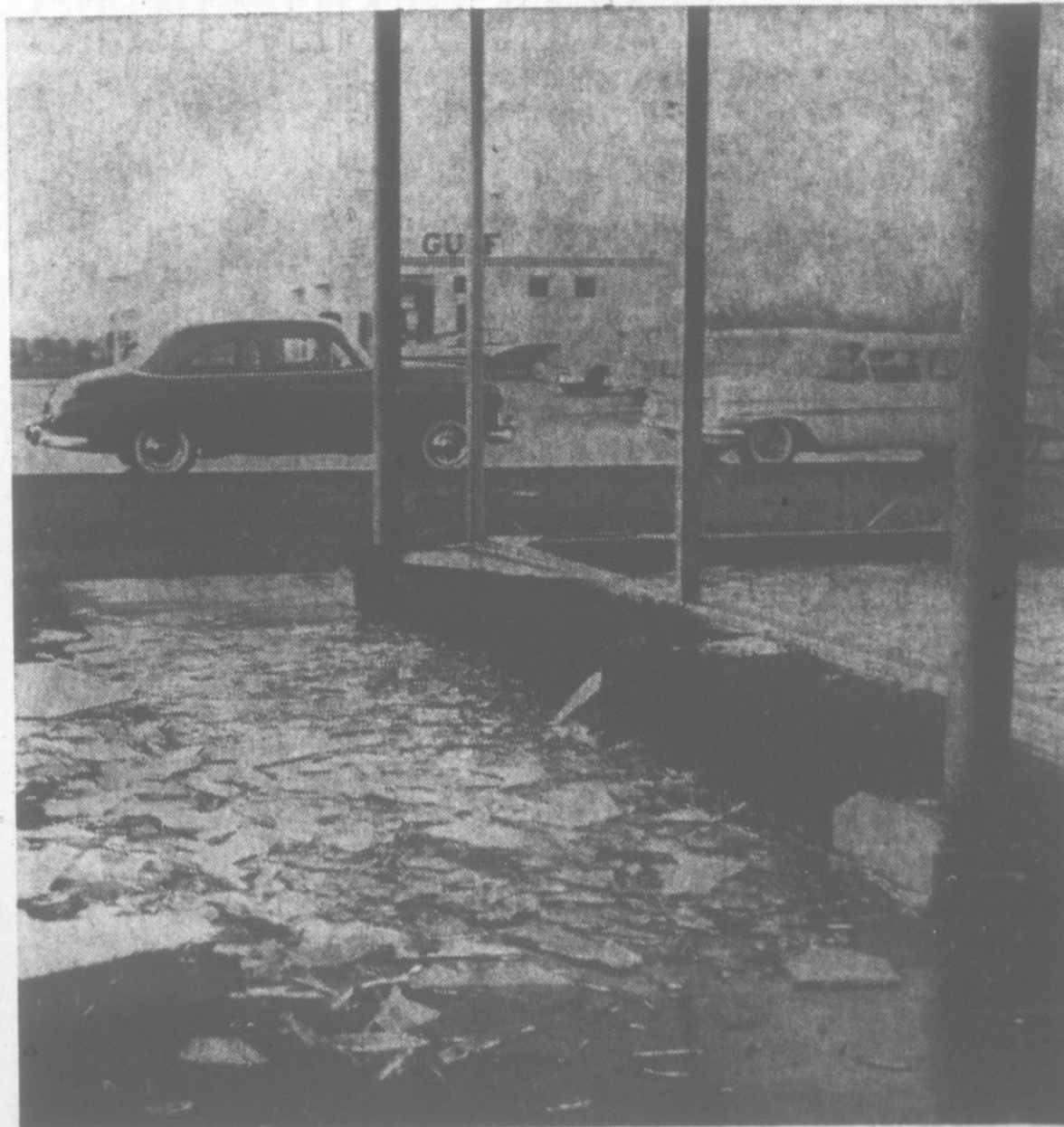
BROKEN GLASS . . . broken out by high winds last night at White Chevrolet Company on South Dickinson Ave.
