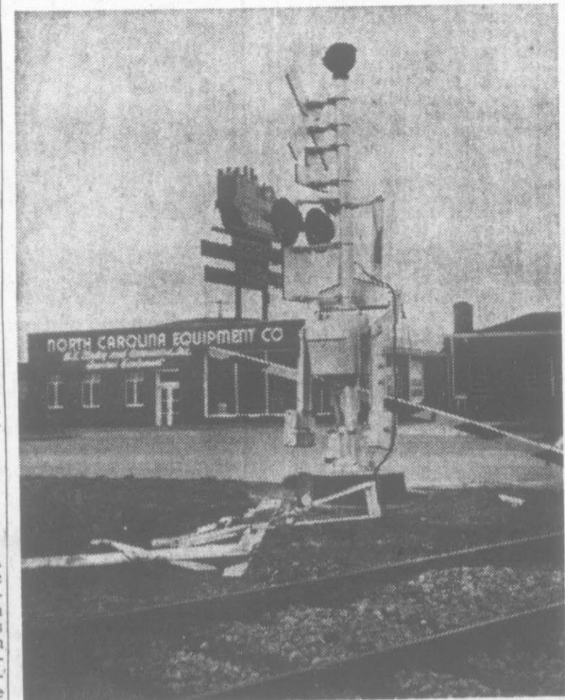
RAILROAD CROSSING BARCADE . . . broken off during storm.
